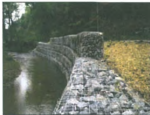
Photo 7.2-12 Gabion baskets can be used for bank stabilisation.
