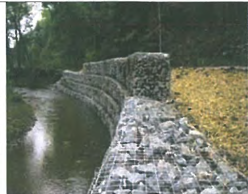
Photo E.5.1-25. Gabion baskets are more durable.
