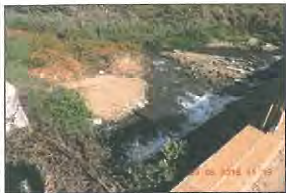
Photo E.5.1-28. Sedimentation observed within the Mofolo Park section of the WMU.
