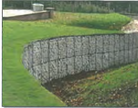
Photo 7.2-14 Box gabions can be used to stabilise river banks.
