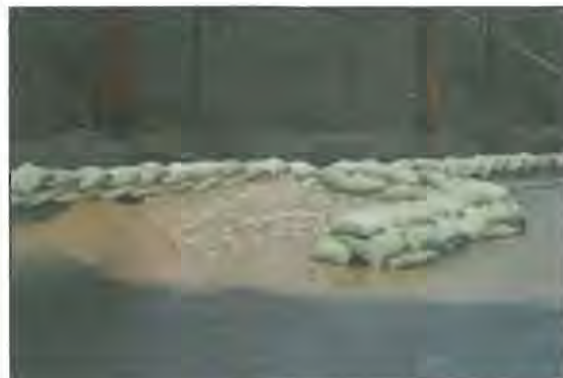
Photo E.5.1-29. Proposed use of gravel bags to combat sedimentation
