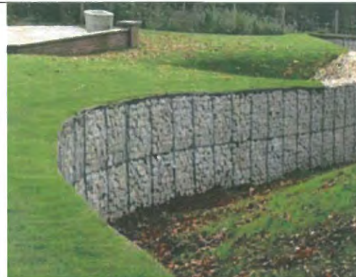
Photo E.5.1-21. Box gabions can be used to stabilise river banks.
