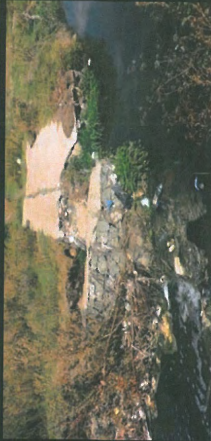
Collapsed gabion
