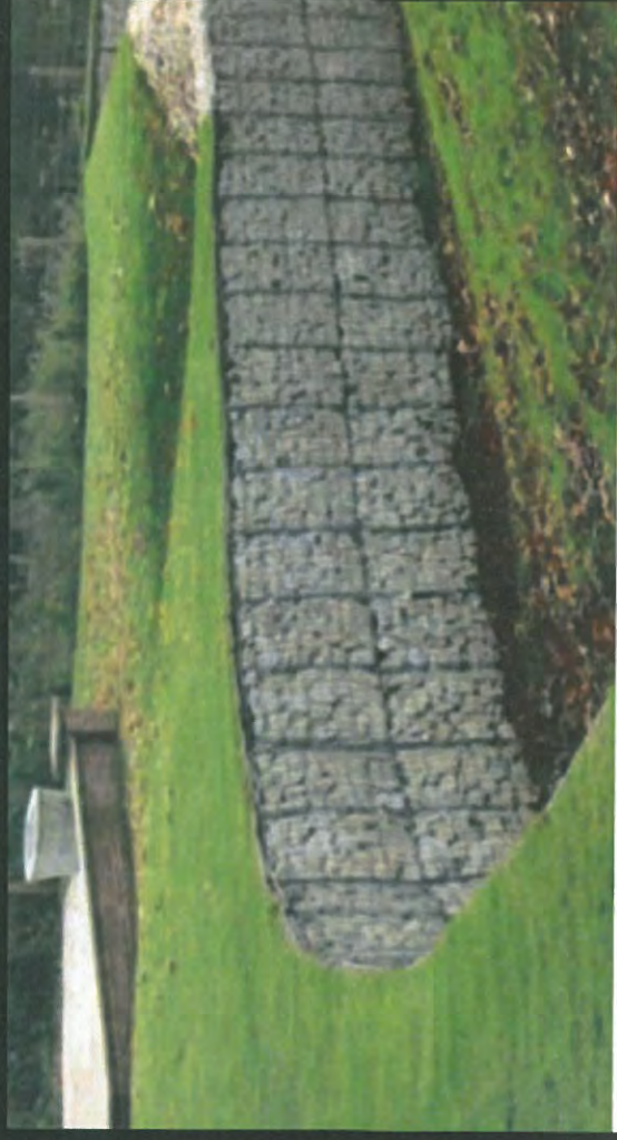
Box gabions can be used to stabilise river banks
