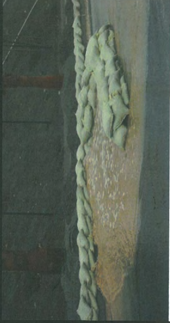
Use of gravel bags to combat sedimentation
