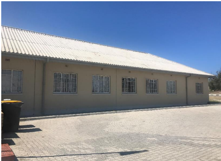
Administration Block buildings
