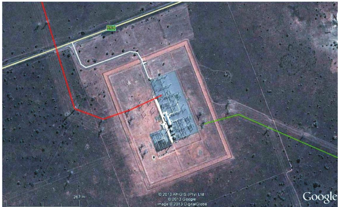
Figure 2. Aerial view of the affected area and substation.
