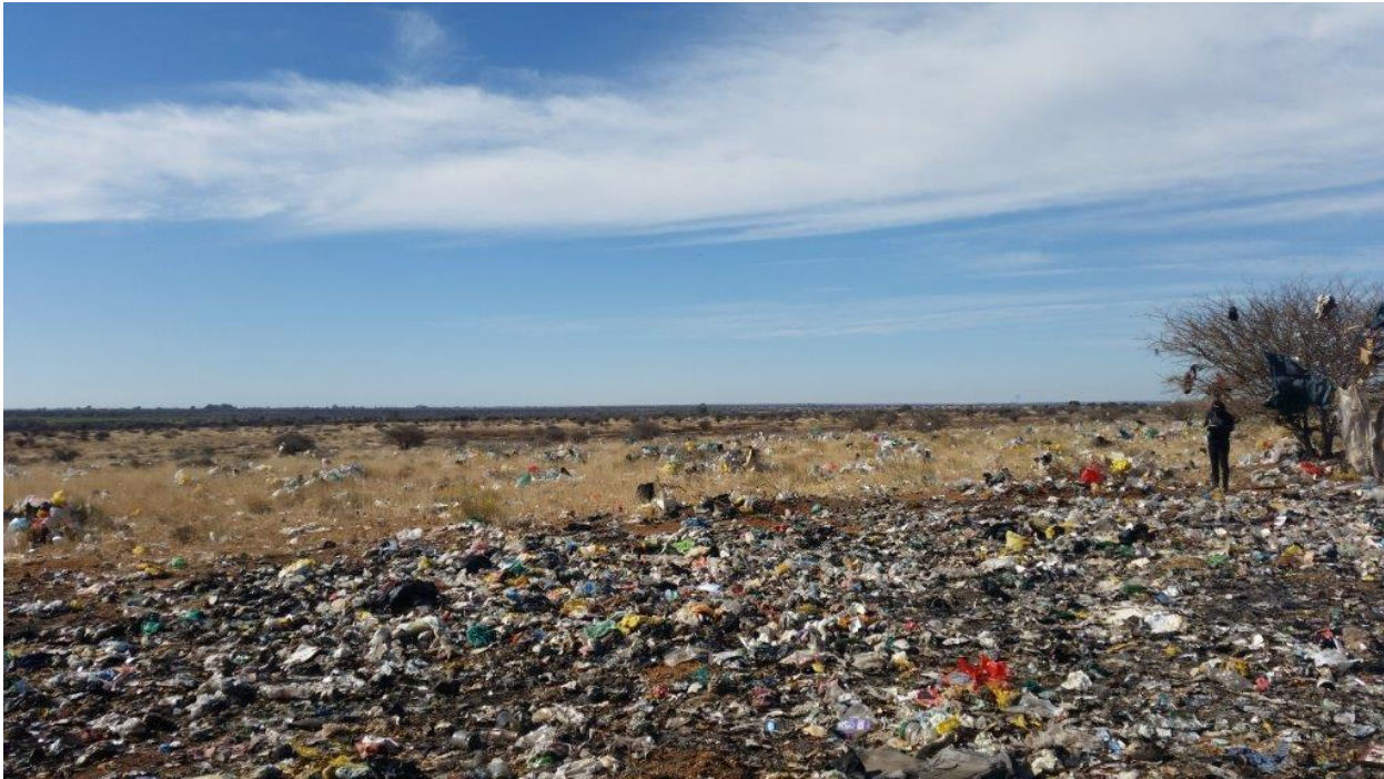
Photoplate 1.3: The south western boundary of the landfill site, note the wind blown litter noted extending to about 700 m from the landfill boundary
