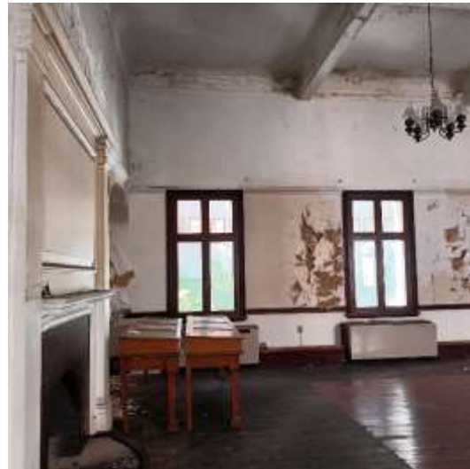
Fig 21 : First floor – Art Gallery – another view
