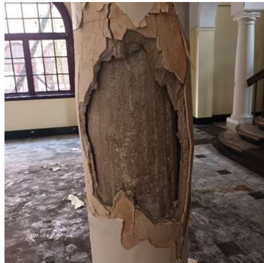
Fig 8 : Exposed concrete column
