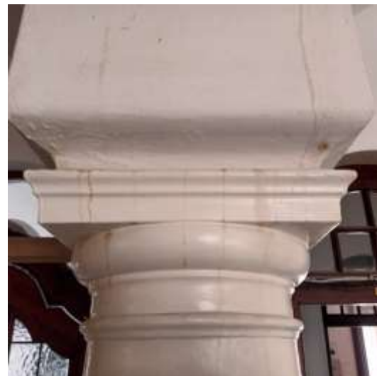
Fig 6 : Top of column
