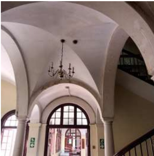
Fig 11 : First floor ceiling
