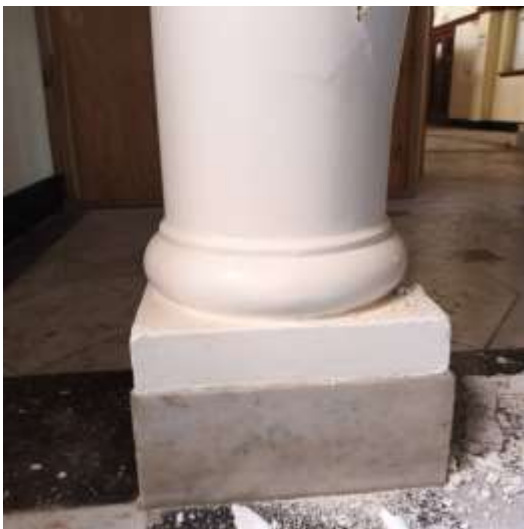
Fig 5 : Typical column base with marble tile cladding
