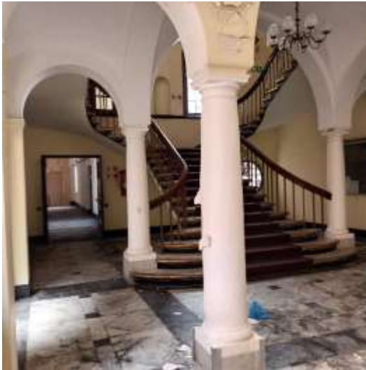
Fig 7 : Ground floor columns around the stairs
