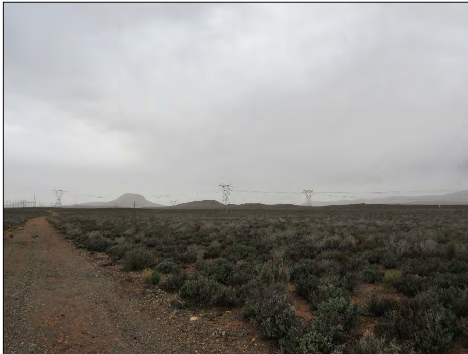
Figure 22: View of high voltage power lines which traverse the study area.
