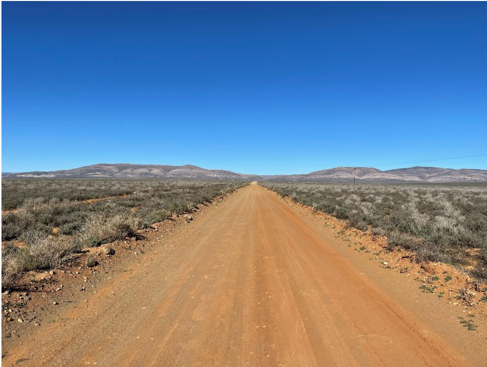
Figure 7.5 Existing Road OP06121 – South Approaching
