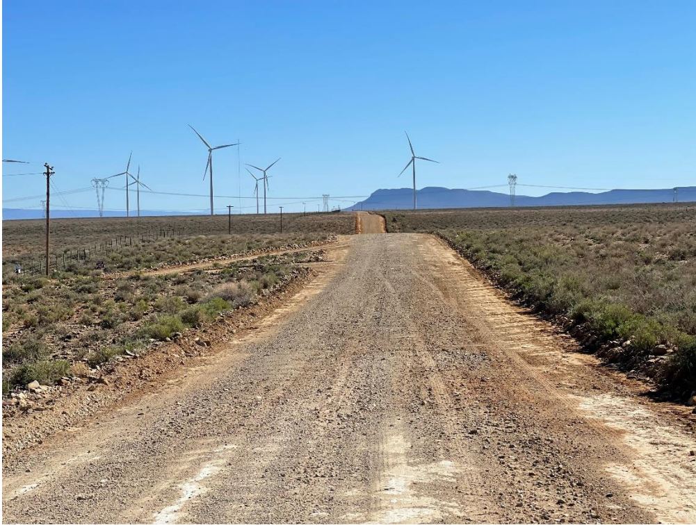
Figure 7.10 Road DR01475 West (Between Km 46.60 – Km 50.73)
