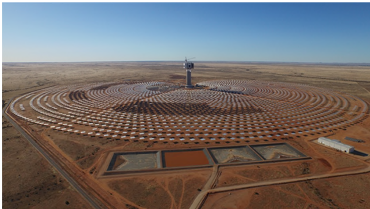
Figure 2.7: Photograph illustrating one of Abengoa Solar’s CSP tower plants close to Upington in the Northern Cape, courtesy of Abengoa Solar S.A.
