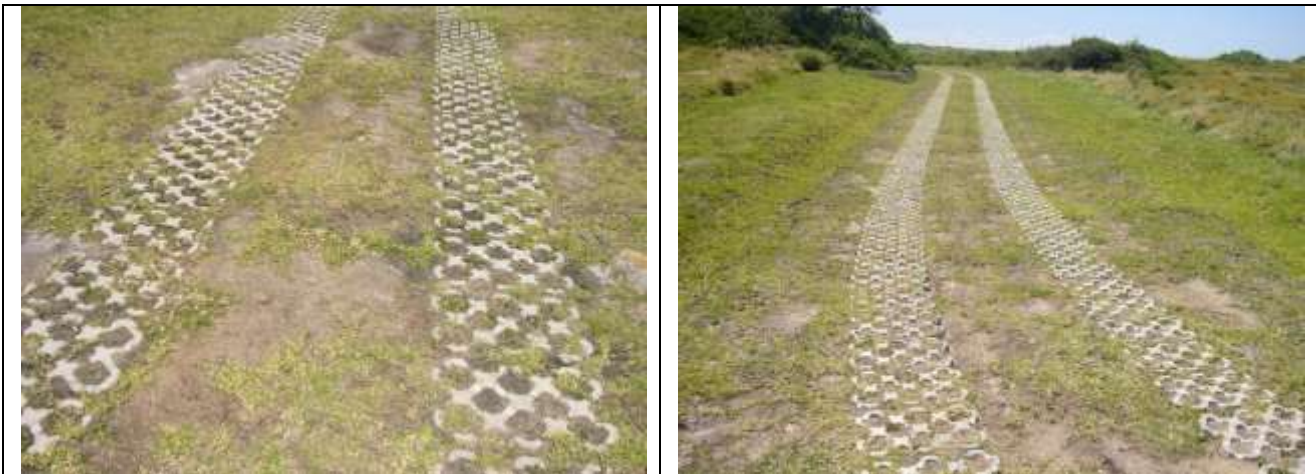
Figure 7.1 Illustration of turfstone eco bricks recommended for the construction of access roads.
