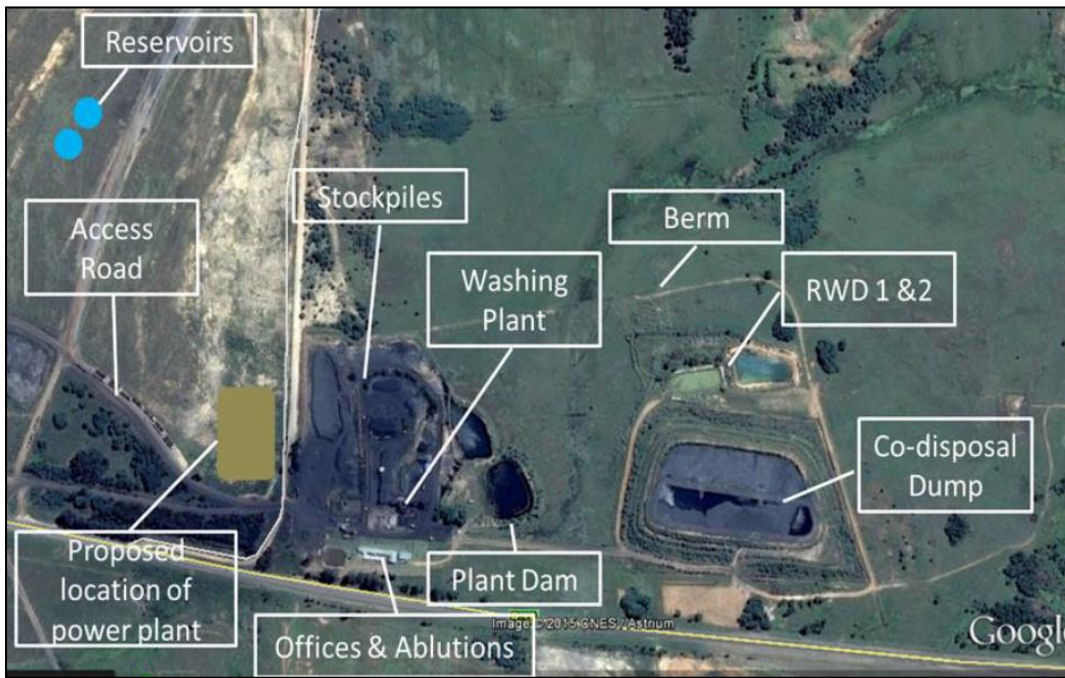
Figure 19: Imbani Wash Plant
