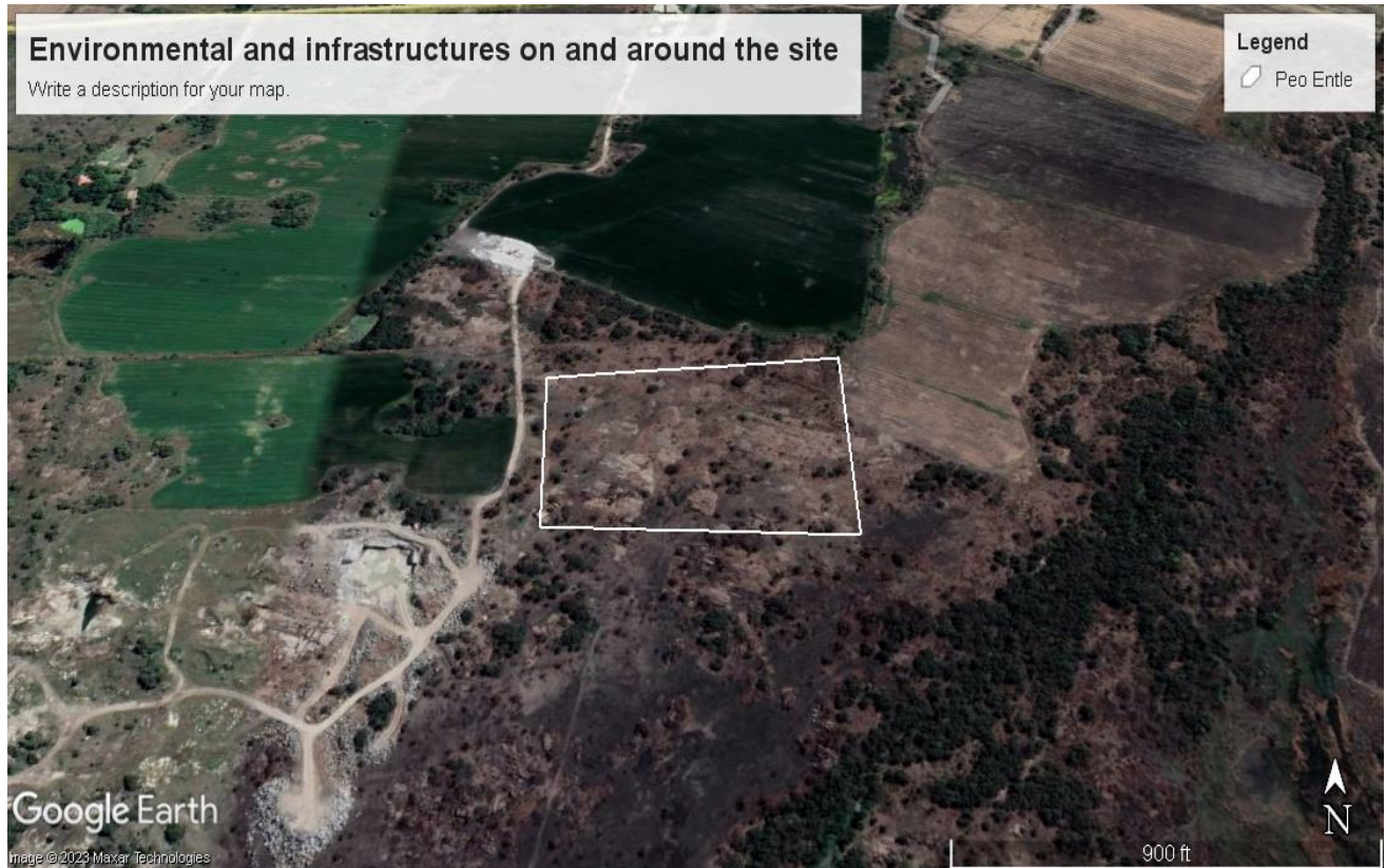
Figure 13: Image depicting the various infrastructures close to the application area mainly agricultural activities (green areas).
