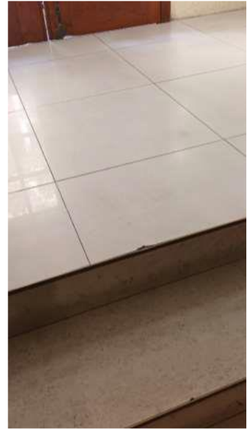
Figure 8 Broken Tiles
