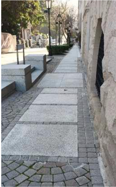
Figure 6 Ramp to Entrance
