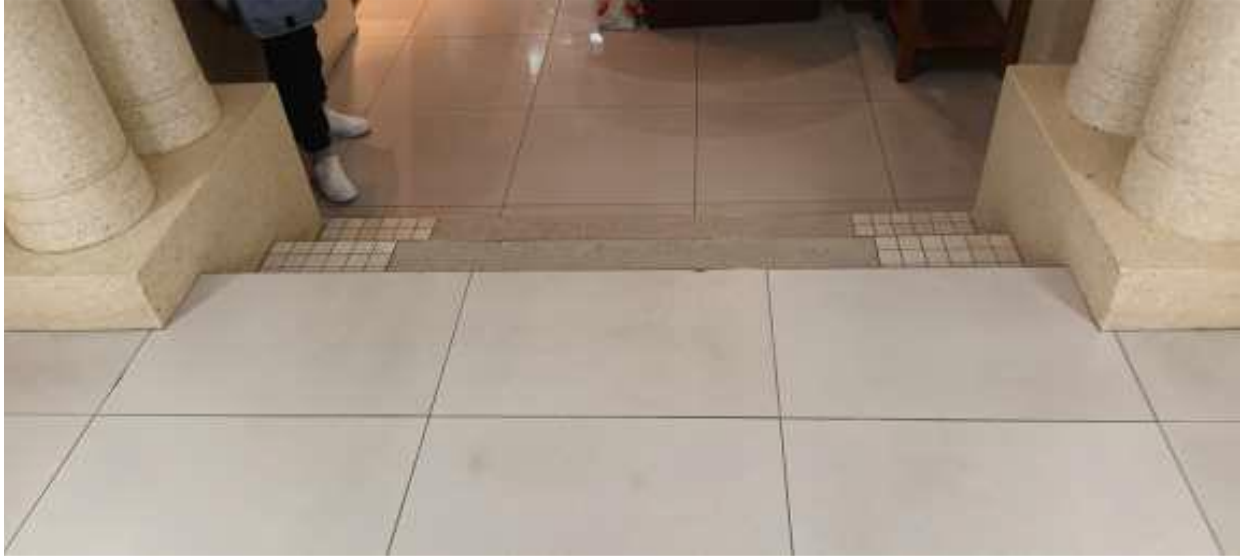
Figure 10. Main Entrance: Distance between steps and security desk
