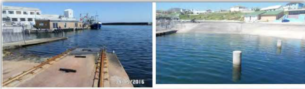
Figure 6: Slipway 1 (left) and Slipway 2 (right)
