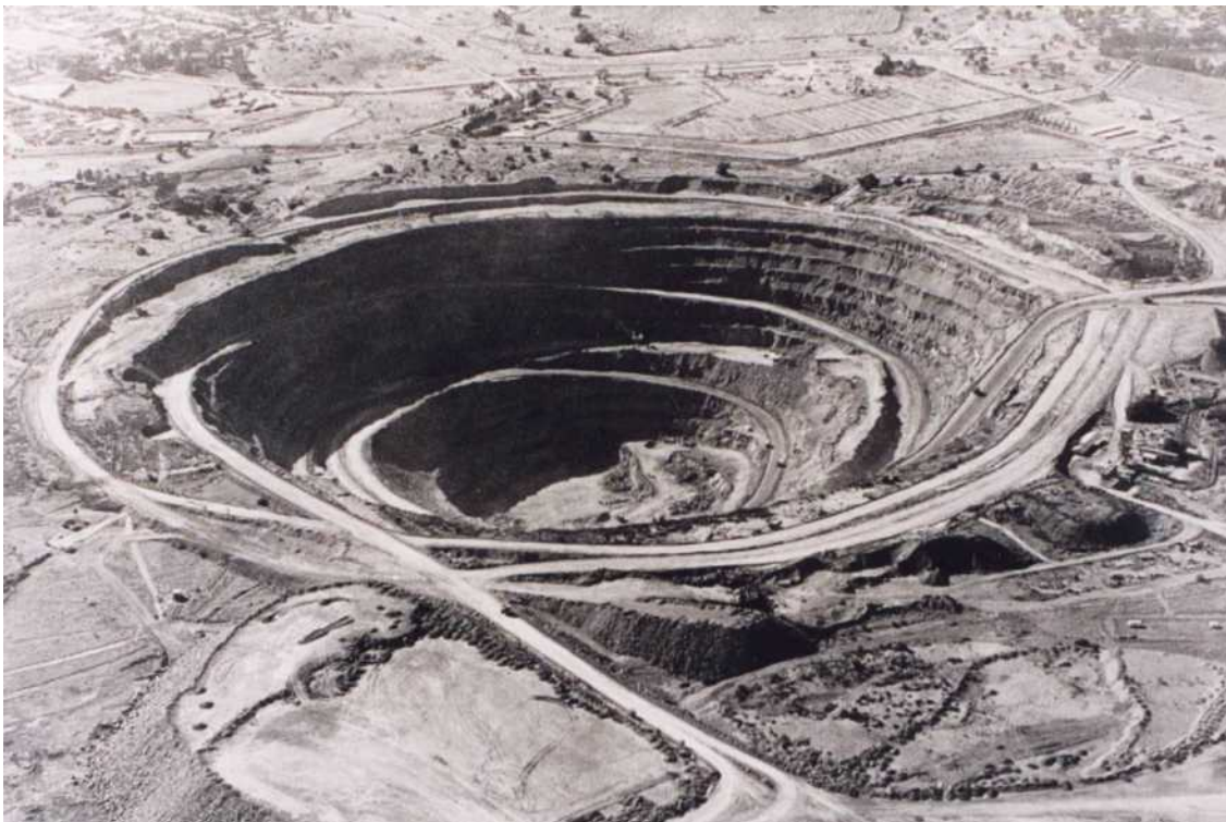
Figure 4. Photograph taken in 1970 of the Koffiefontein pipe during construction of the mine shaft for underground mining. The Whitworth Dump is visible on the far side of the pipe.
