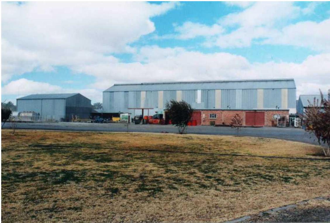
Figure 148. Building now standing where graves were located
