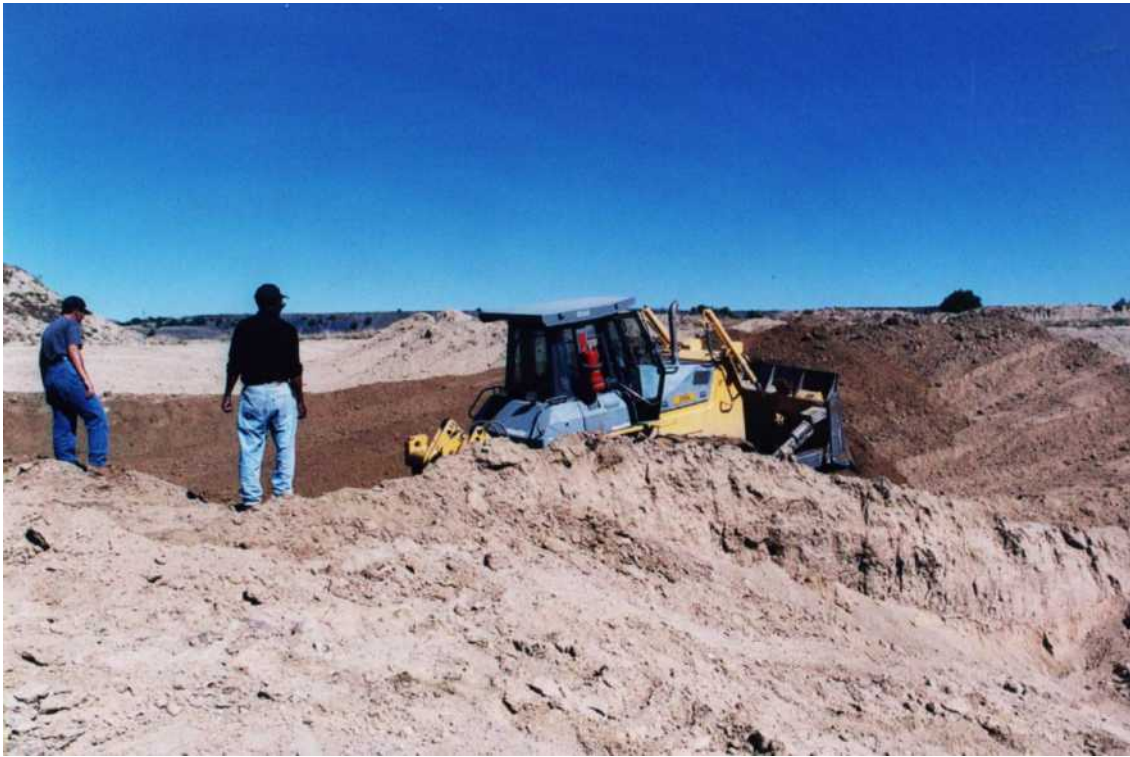
Figure 11. Bulldozing in progress.
