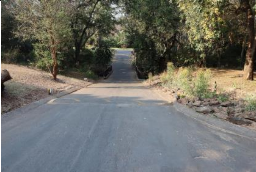
Road crossing bisects riparian area
