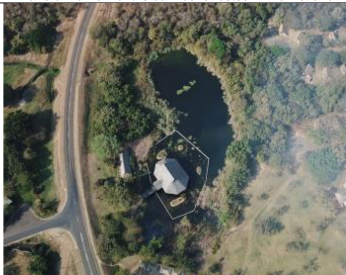
Aerial photo indicating the extent of the dam
