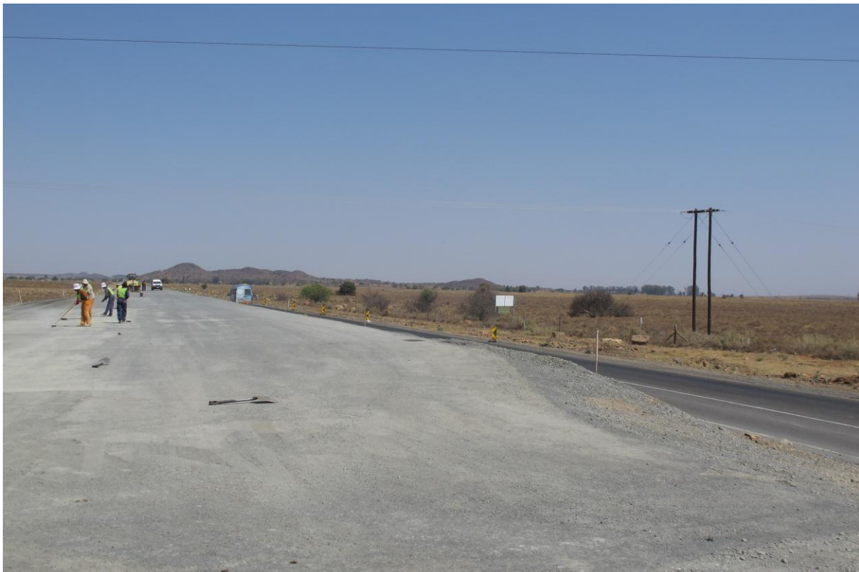
Image 20: N8 national road construction
