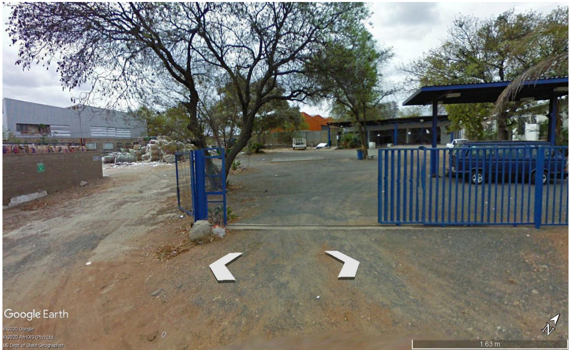
Figure 1-2 Entrance to filling station
