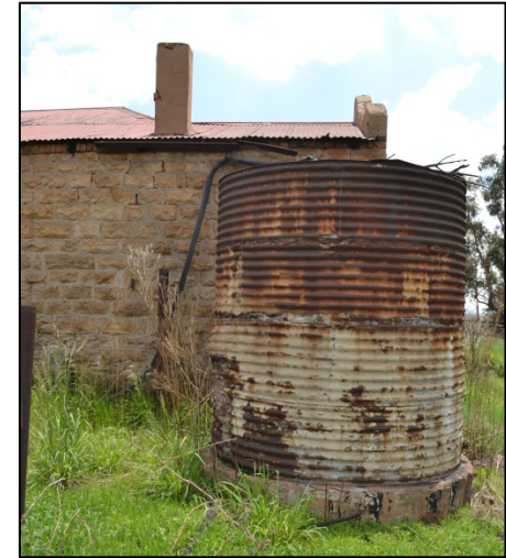
Figure 43. Down piping was discarded and water from the gutter flowed directly into a water reservoir (Photograph: M. Naude 2016).
