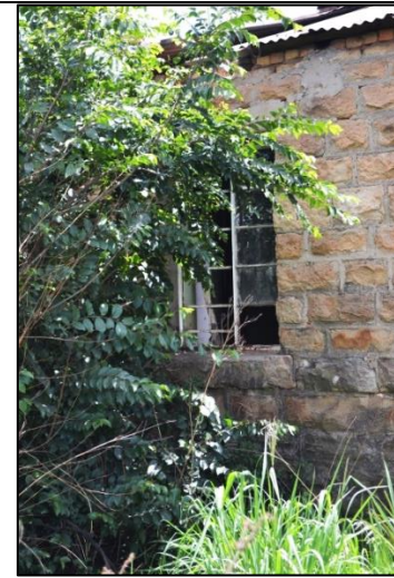
Figure 35. Steel frame window in the southern elevation (Photograph: M. Naude 2016).
