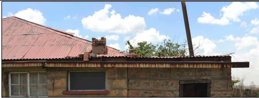
Figure 42. Box gutter along the western elevation and extension (Photograph: M. Naude 2016).
