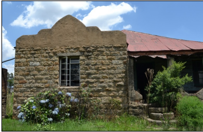
Figure 5. Front facade with gable room executed in dressed sandstone with the parapet front gable done in plastered brick (Photograph: M. Naude 2016).
