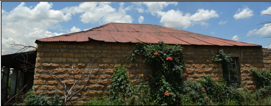
Figure 21. General condition of the corrugated sheet iron roof (Photograph: M. Naude 2016).
