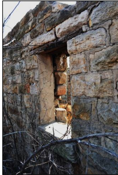
Figure 20. Window with timber lintel intact
