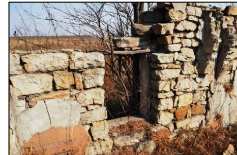
Figure 21. Small window with remnants of the timber lintel at the top
