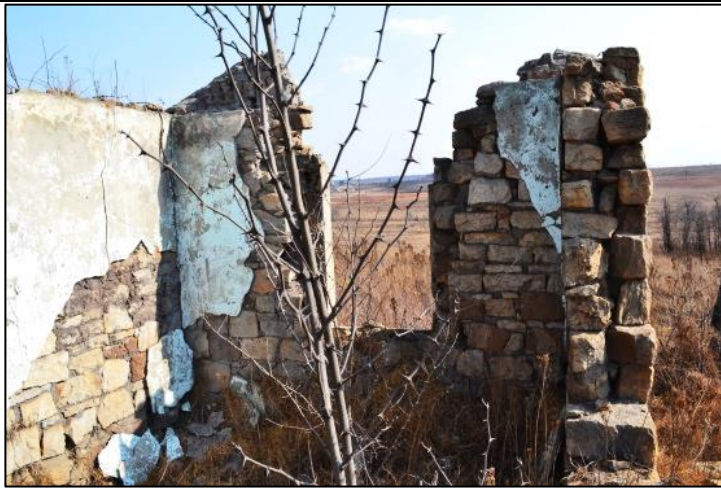
Figure 9. Exposed stone masonry walling of the gable
