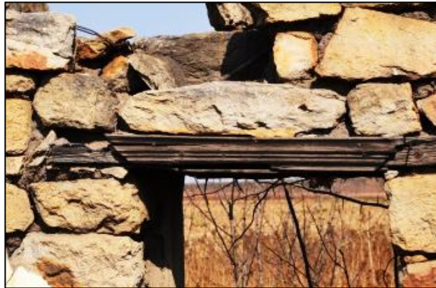
Figure 19. Window with lintel and architrave intact
