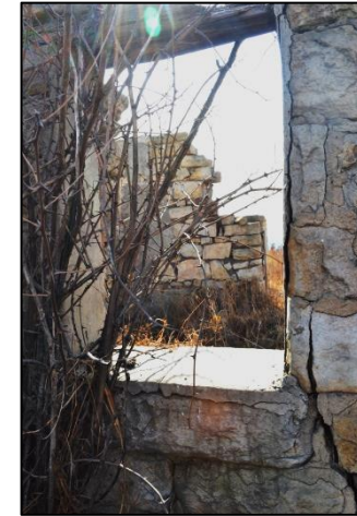
Figure 23. Window with solid sandstone window sill
