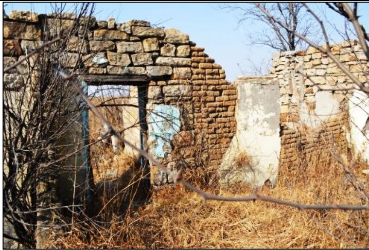
Figure 7. Part of the exterior walling with clay bricks forming part of a later addition
