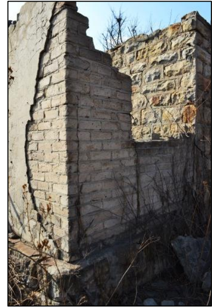
Figure 22. Well-prepared sundried clay bricks used for this recent addition exposed after the plastered was broken and had fallen off
