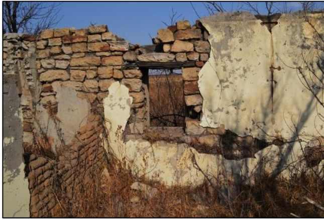
Figure 18. Window with lintel and a short section of the top part of the architrave intact
