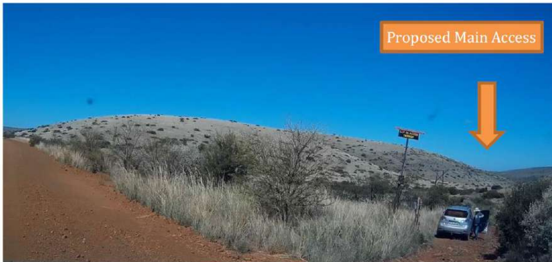
Figure 2.6: Main access to Kuruman WEF (Phase 2) via D3420.
