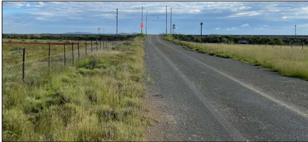
Figure 9: Burgerville Gravel Road
