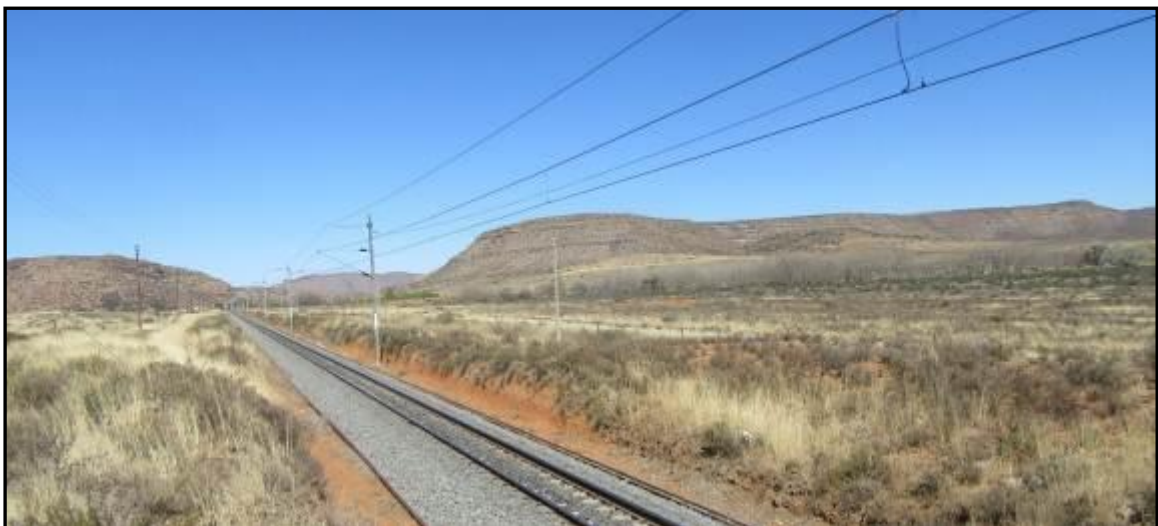
Photograph 7.7: Railway line and 132 kV transmission line on Edendale north of farmyard
