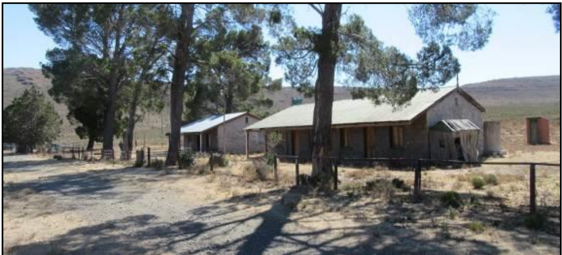
Photograph 7.5: Cottages associated with former De Rust siding on non-site portion of De Rust
