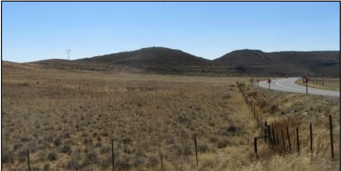
Photograph 7.12: N9 and 132kV line across north-eastern portion of Vrede
