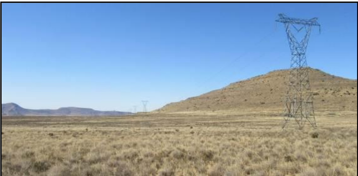
Photograph 3.20: Existing 132 kV line across south-western portion of De Rust
