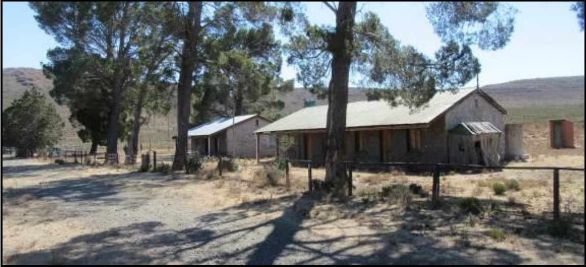
Photograph 3.19: Cottages associated with former De Rust siding on non-site portion of De Rust
