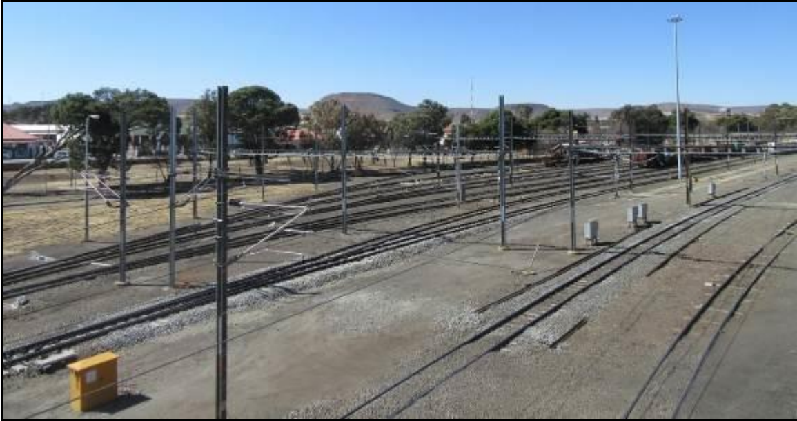
Photograph 3.4: Noupport station seen from the train bridge in Noupport
