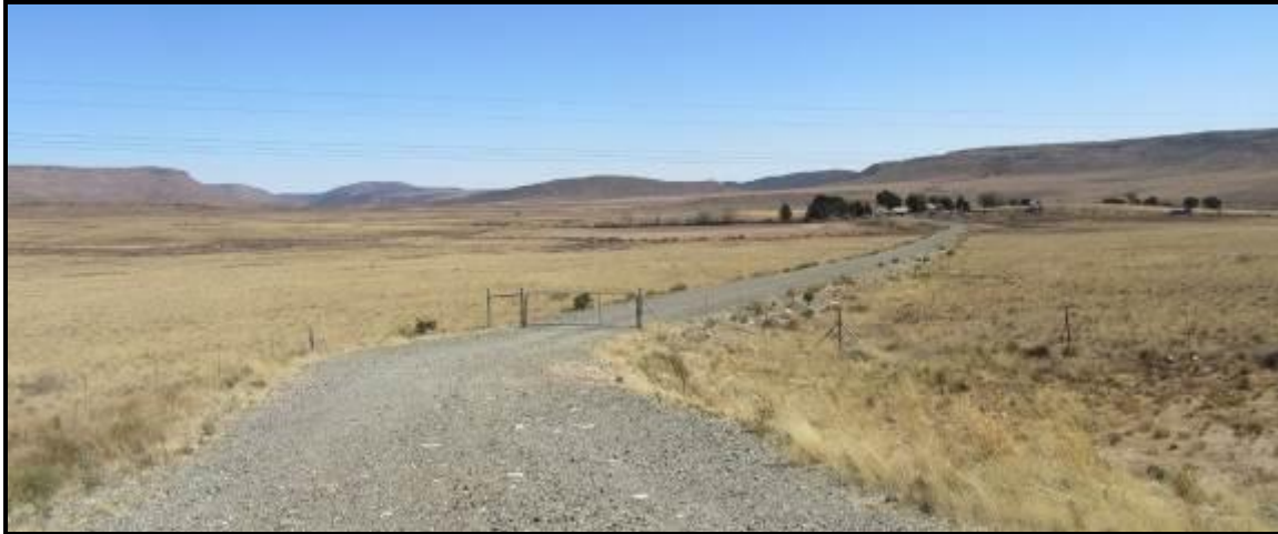
Photograph 3.24: Vrede farm yard and access road off the N9. Note 132 kV cables traversing access road in foreground
