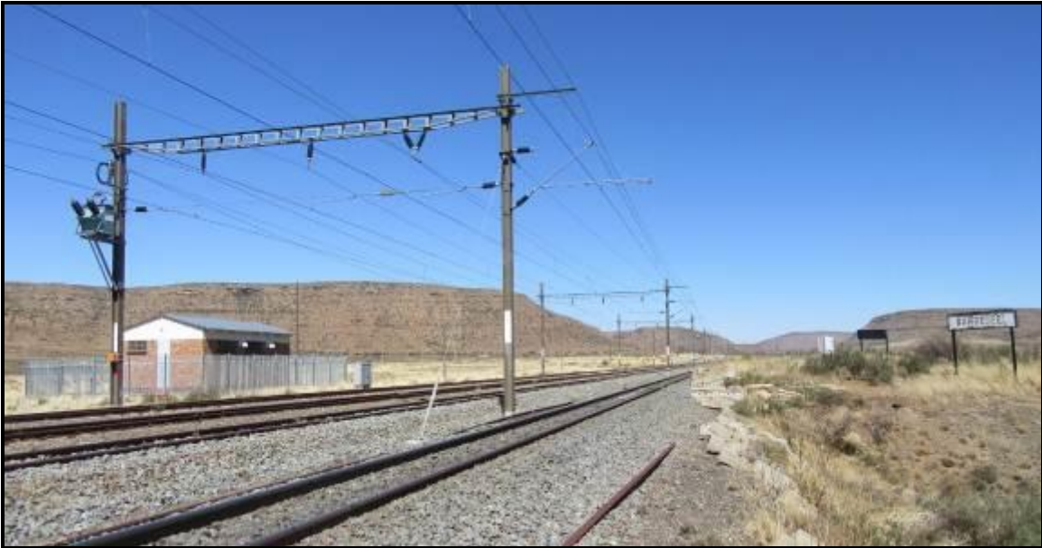
Photograph 3.14: Barredeel siding located to the west of the N9 north of Edendale. Turbines are proposed on the ridgeline to the left of the line (Hartebeeshoek)
