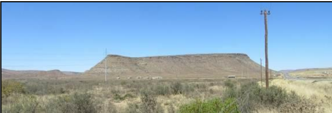
Photograph 3.30: Noupoort WEF 132 kV feeder line across site portion of Hartebeeshoek. The defunct broiler farm is in the middle distance, N9 to the right
