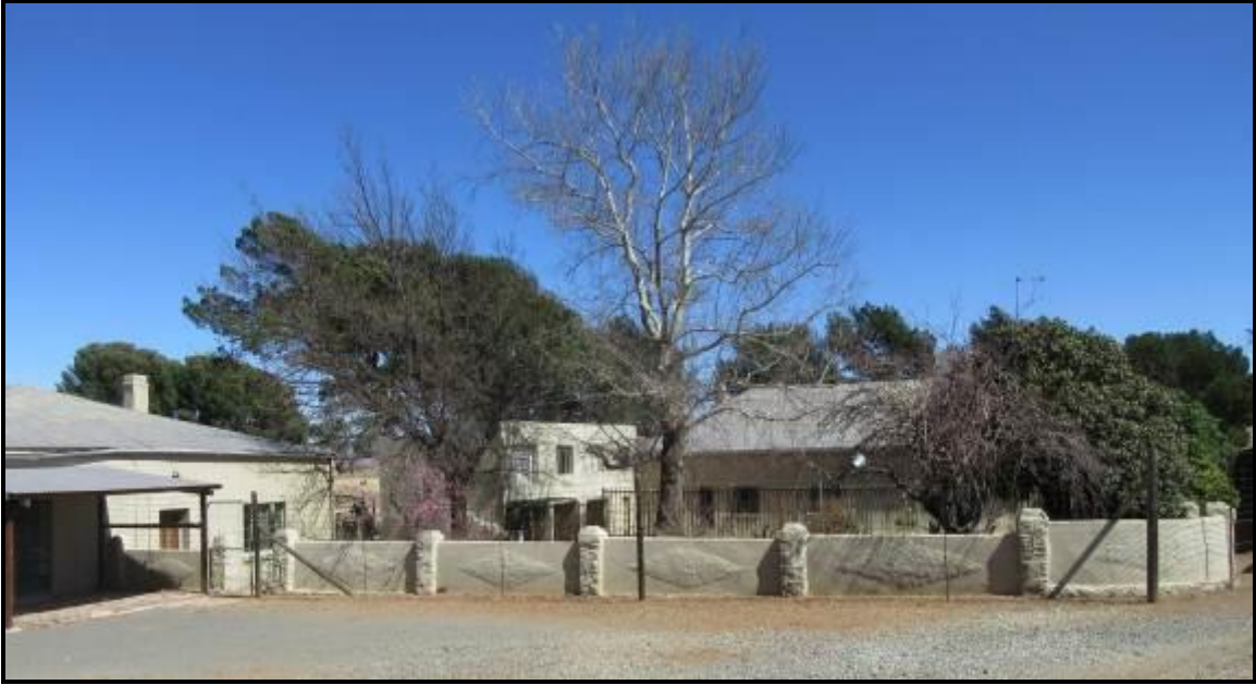
Photograph 3.25: Uninhabited farm house and out buildings on Vrede
