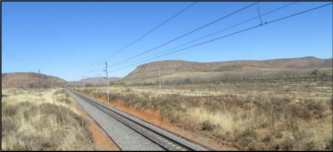
Photograph 3.21: Railway line and 132 kV transmission line on Edendale north of farmyard
