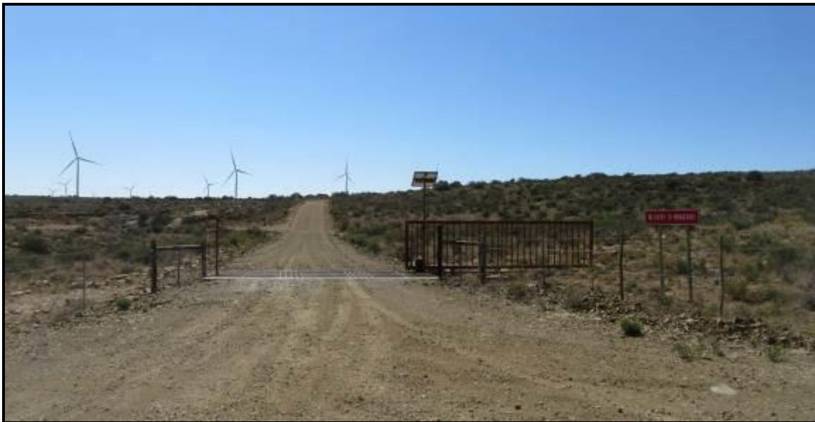
Photograph 3.42: One of two entrances to the Noupoort WEF off the Oorlogspoort gravel road
