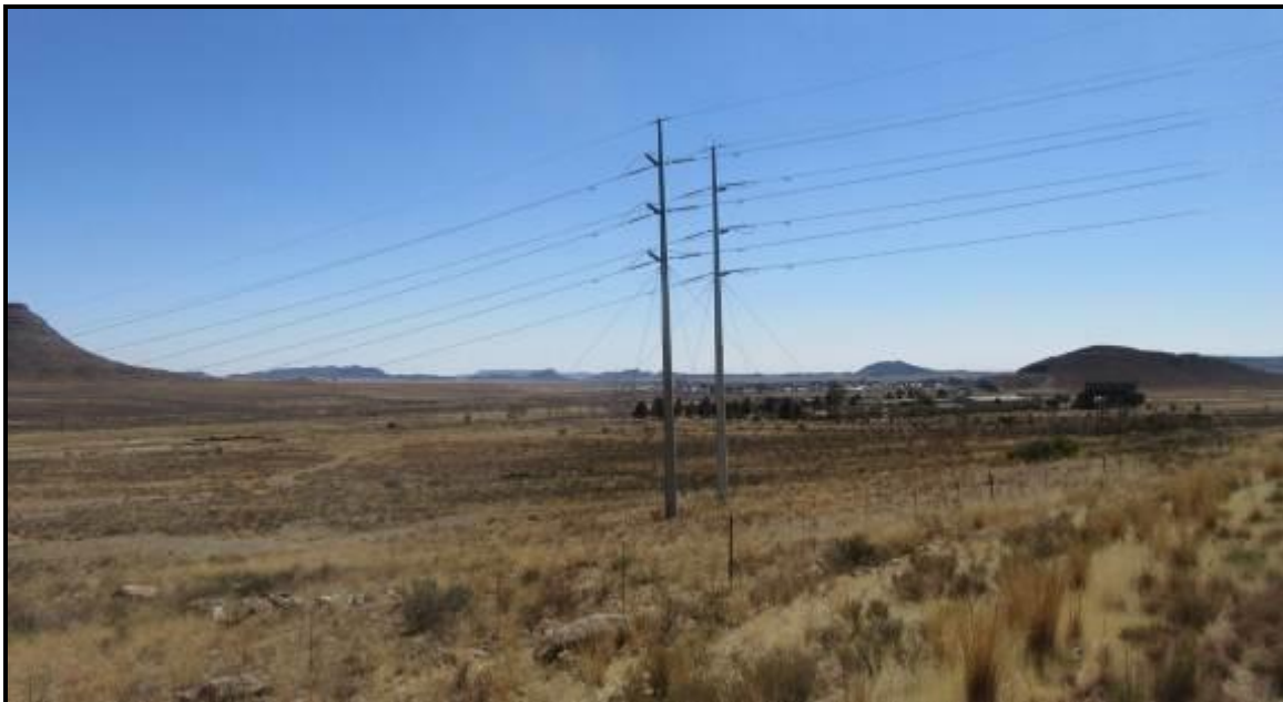
Photograph 3.38: Existing feed in Tx line from the Noupoort WEF which traverses the N9 between Barredeel rail siding and Midlandia.
