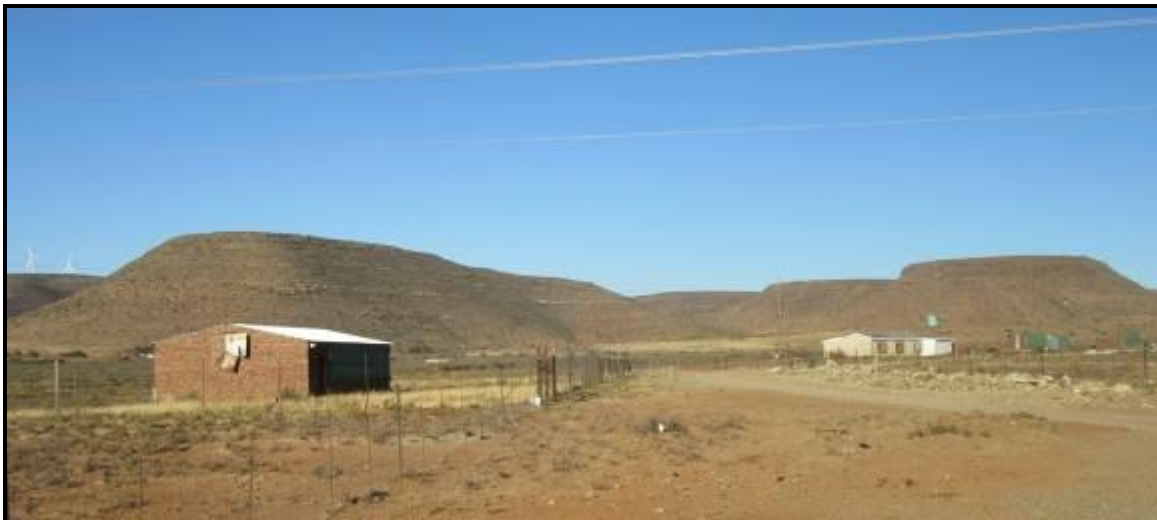
Photograph 3.37: Existing entrance road to Hartebeeshoek off the N9, with buildings of the defunct broiler project on either side
