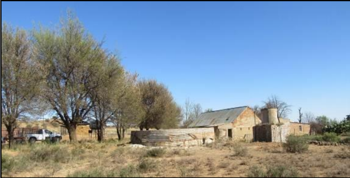
Photograph 3.15: Farm house on Kleinfontein, now used for storage
