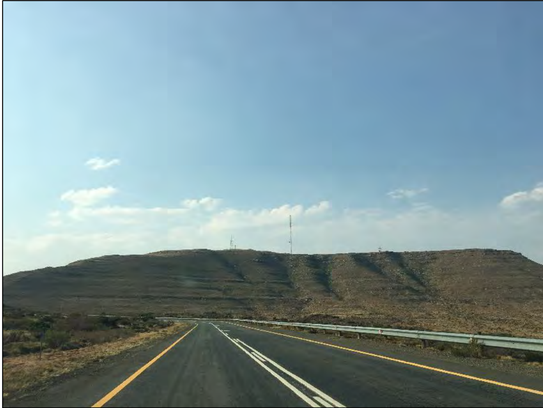
Figure 51: View of some of the typical tall linear anthropogenic elements which can be seen from the N9 and N10 national routes.
