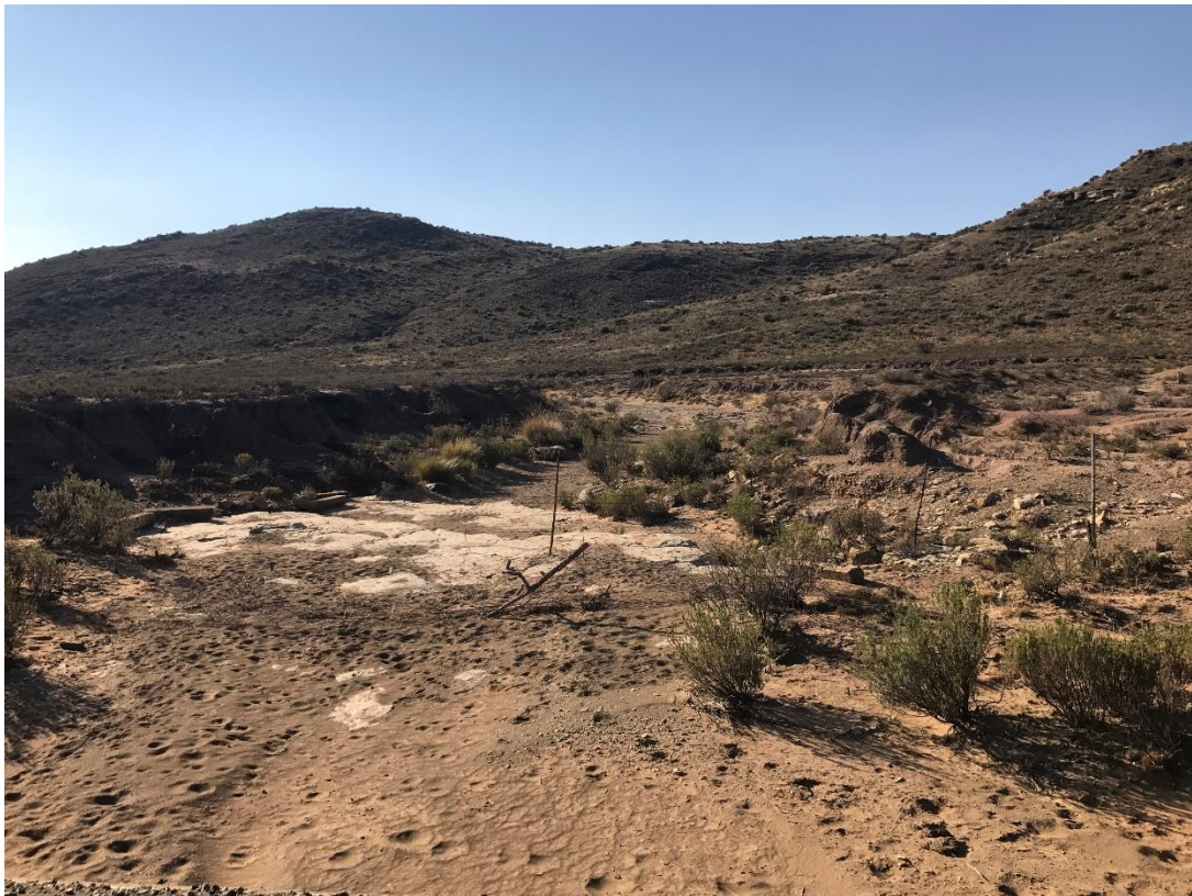
Plate 2: A number of the larger water courses had some form of erosion or head cut formation present
