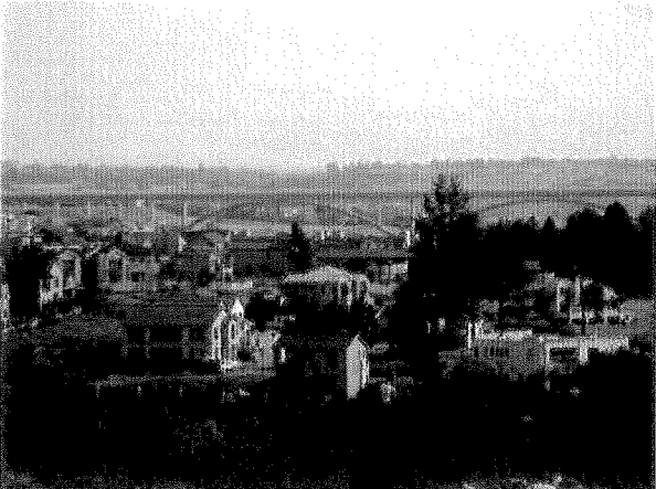
Sewage pipe in urban area
