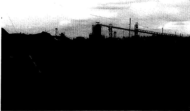
Plate 1-2: Phola Coal Processing Plant (CONVEYOR START POINT)
