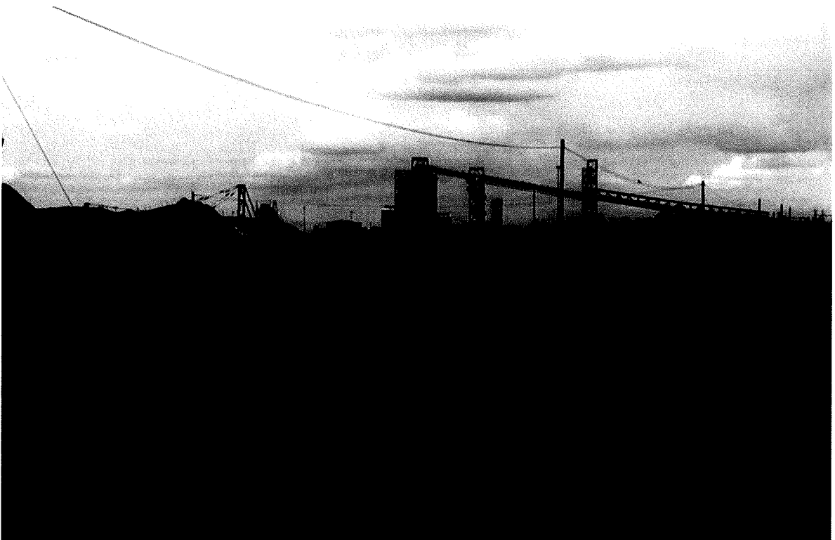
Plate 1-2: Phola Coal Processing Plant
