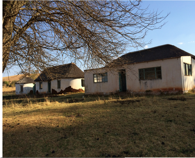
Doornek picket to be demolished
