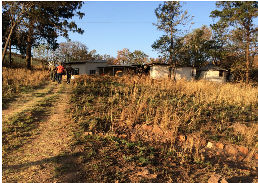
Hondekraal gate picket to be demolished
