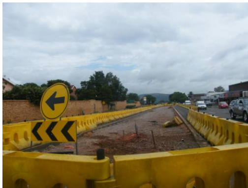
Photograph 11: BRT construction activities on the western side of the site
