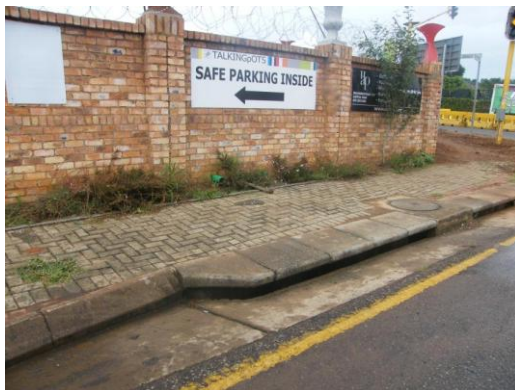
Photograph 6: The fenced proposed site from Malherbe Street
