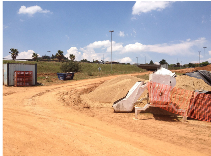
Looking South-East from middle of site
