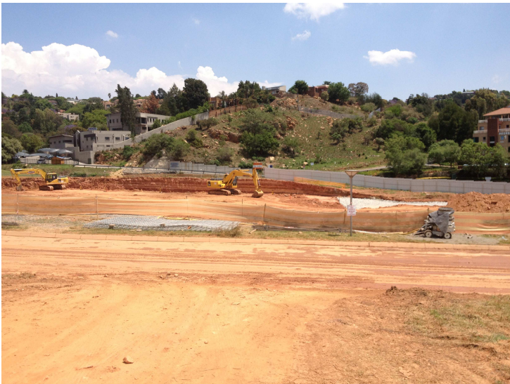
Looking West from middle of site
