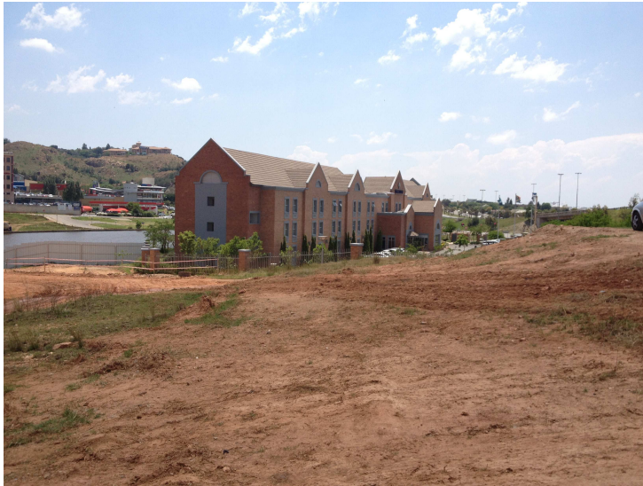
Looking North from middle of site
