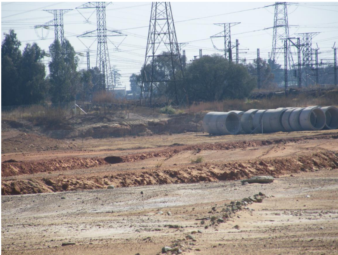
Photograph 6: Looking north from the middle of the site - Randwater pipeline construction
