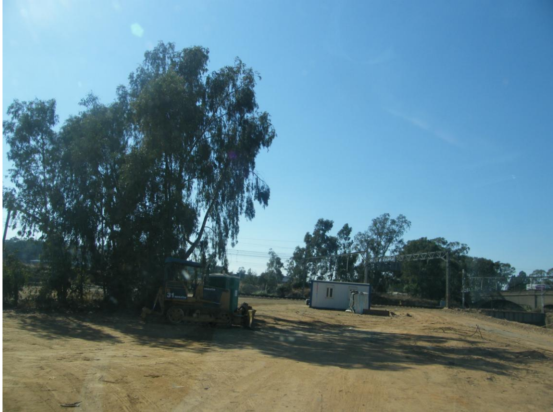
Photograph 16: Transnet site office located at the south-east access to the site
