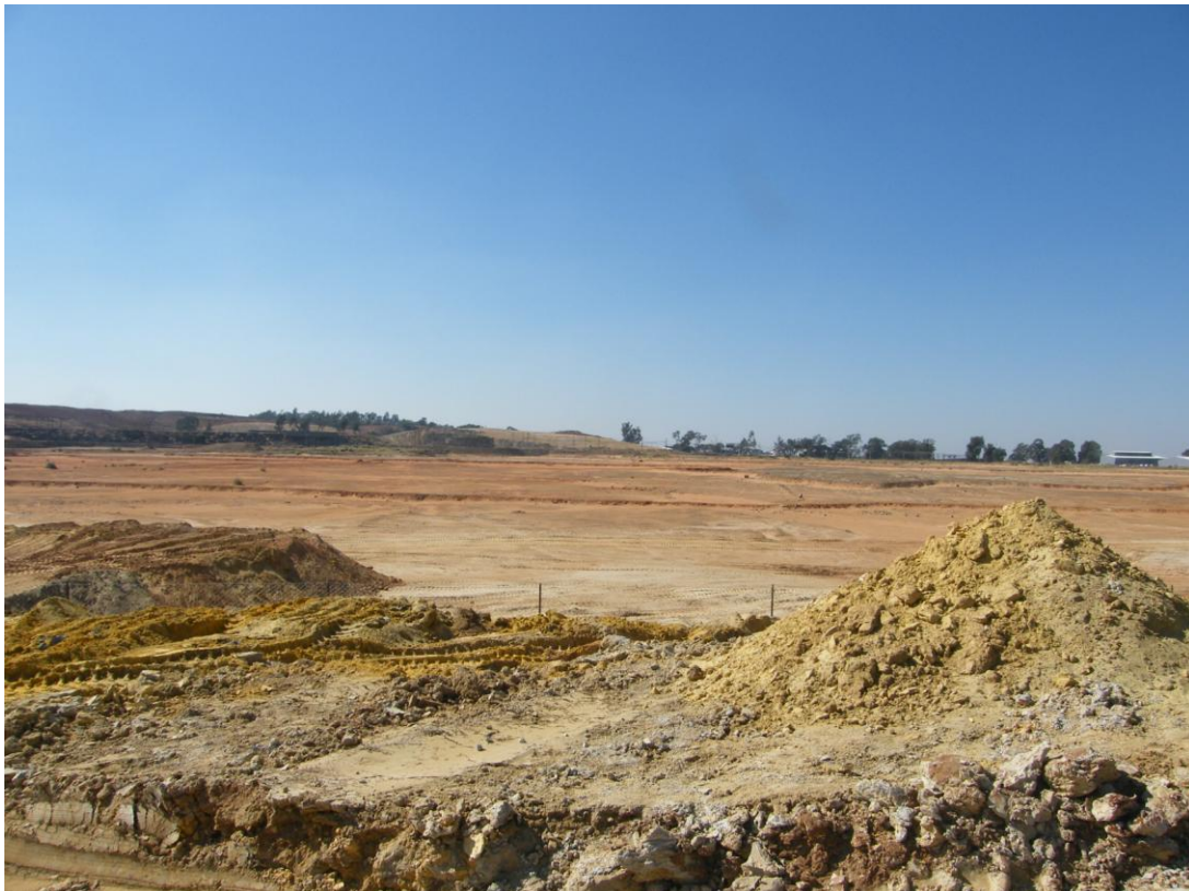
Photograph 10: Soil stockpiles located next to the pipeline construction
