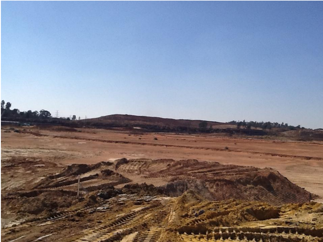
Photograph 11: Looking east from the western border of the site
