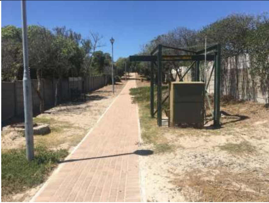
View from the ACE BMH inland. No further disturbance to the terrestrial environment will be required as the 2AFRICA/GERA (East) Cable System will be housed in spare ducts installed when the ACE Cable system was landed by MTN.
