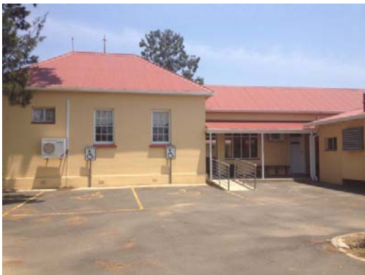
Back of Main Building - Library and Cash Hall with Holding Facility on the right
