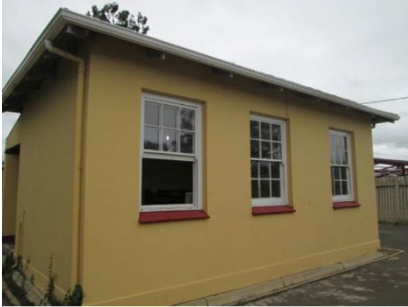
External views of existing Gate House
