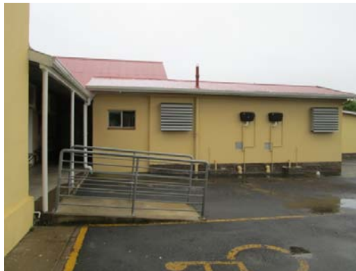
Holding Facility at the back
