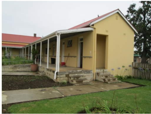
Office wing closest to street
