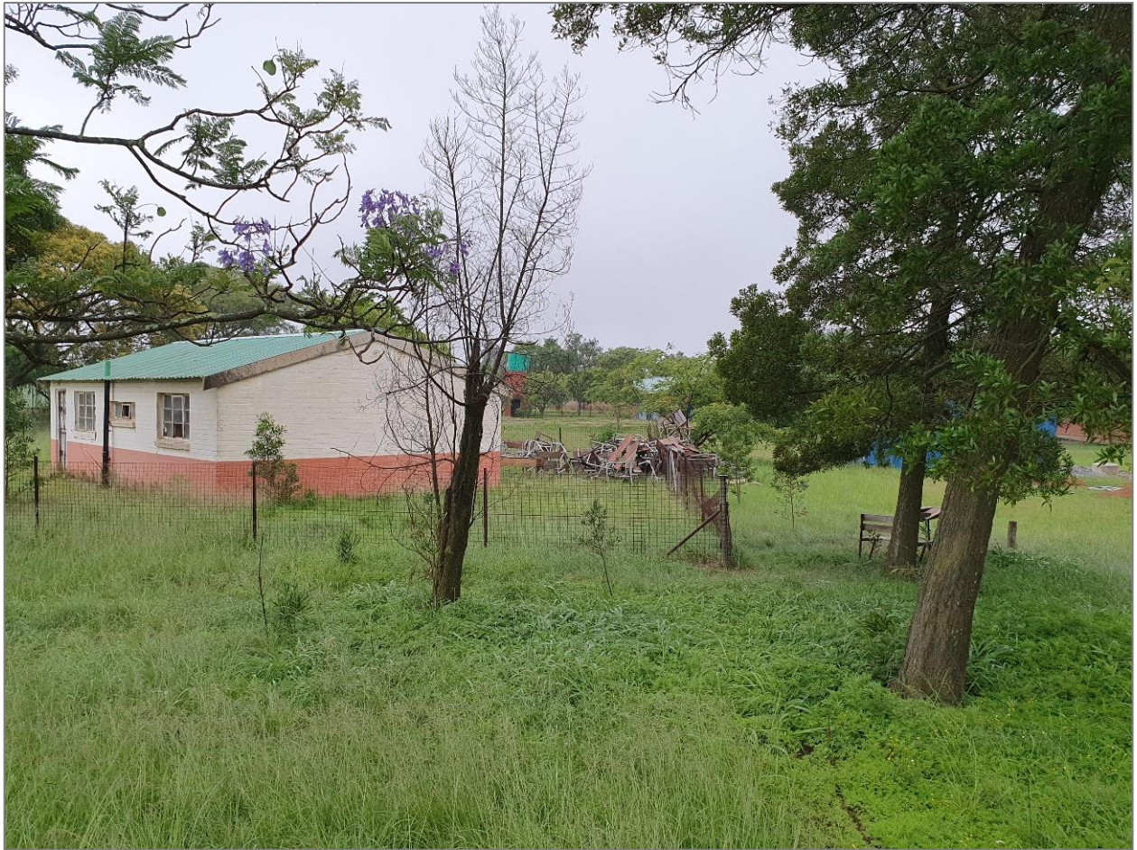
Figure 5: View of proposed development site from south-eastern boundary line (facing northwest). Note: Existing staff residency (Block 10; left-hand side), which is earmarked for demolition and replacement with brick-and-mortar structure.
