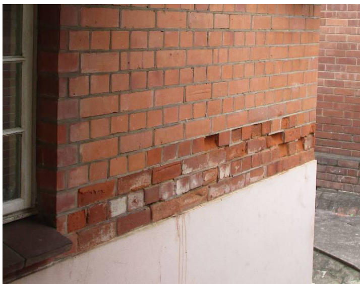
Deterioration of brickwork
