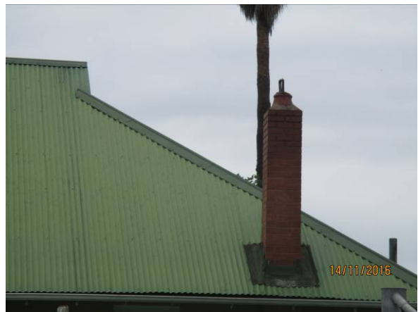
Kitchen Chimney Stack
