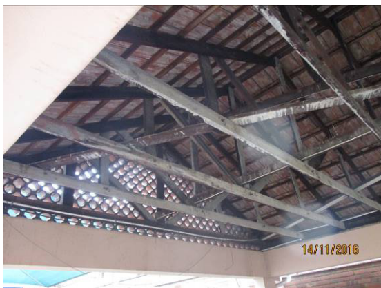
Underside of shaded parking structure
