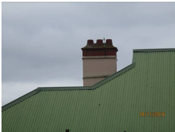
Main Chimney Stack
