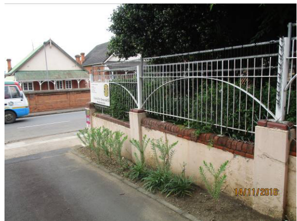
Retaining wall on street
