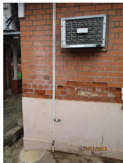
Damaged brickwork
