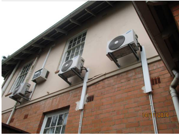
New & old airconditioners (damage to brickwork)
