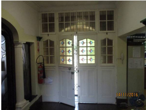
Main Entrance (Internal)
