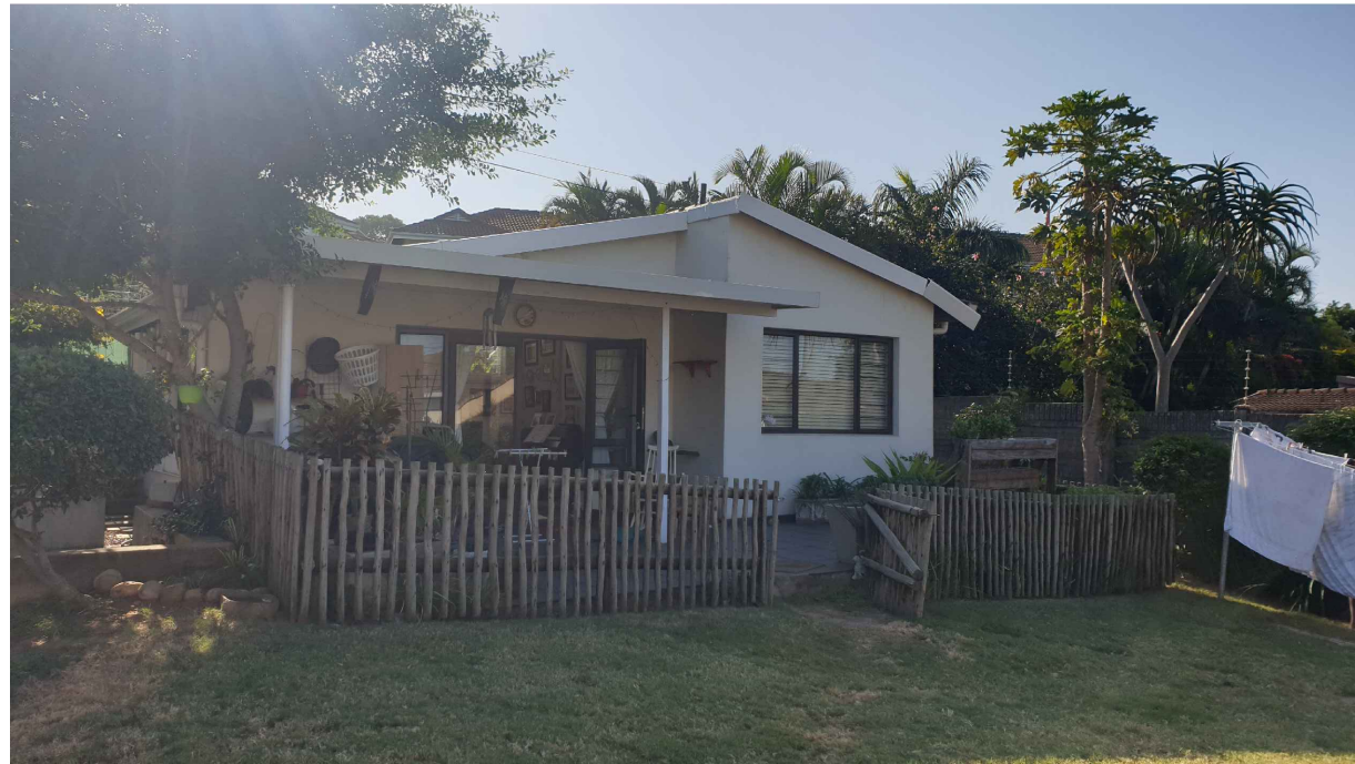
OUTBUILDING SOUTH EAST VIEW
