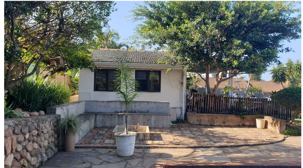
OUTBUILDING SOUTH WEST VIEW
