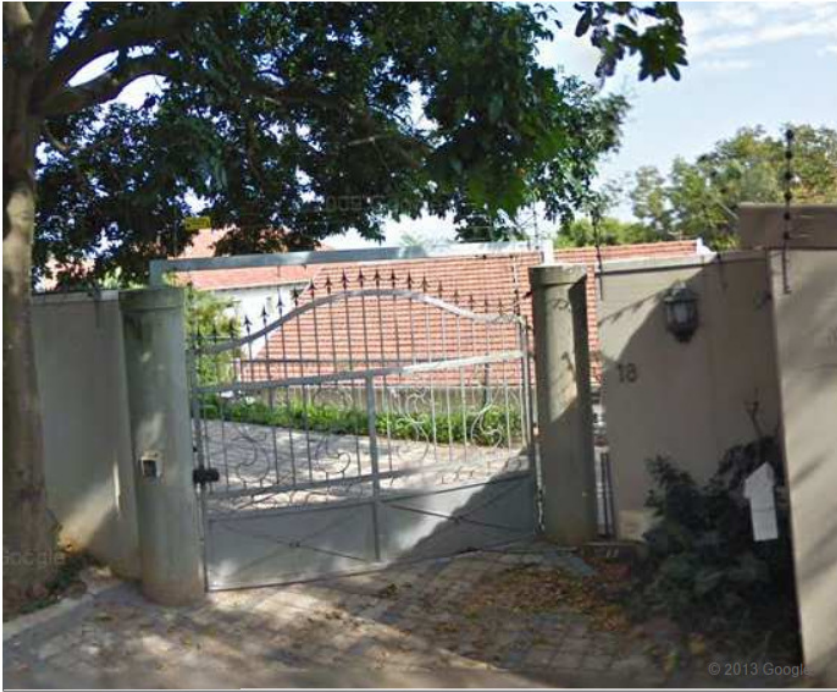
View of entrance gate on Pinsent Road
