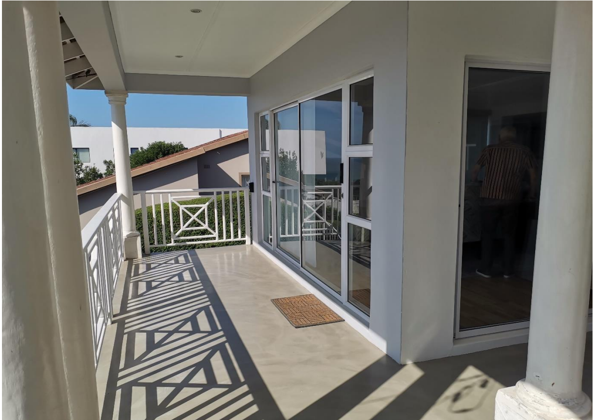
EXISTING COVERED VERANDAH AND SLIDING DOORS
