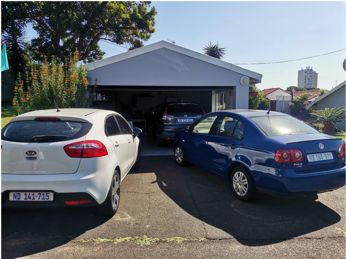
SOUTH ELEVATION OF EXISTING GARAGE
