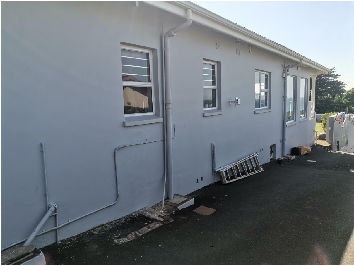
SOUTH ELEVATION CLOSE UP SHOWING NEW AND EXISTING WINDOWS
