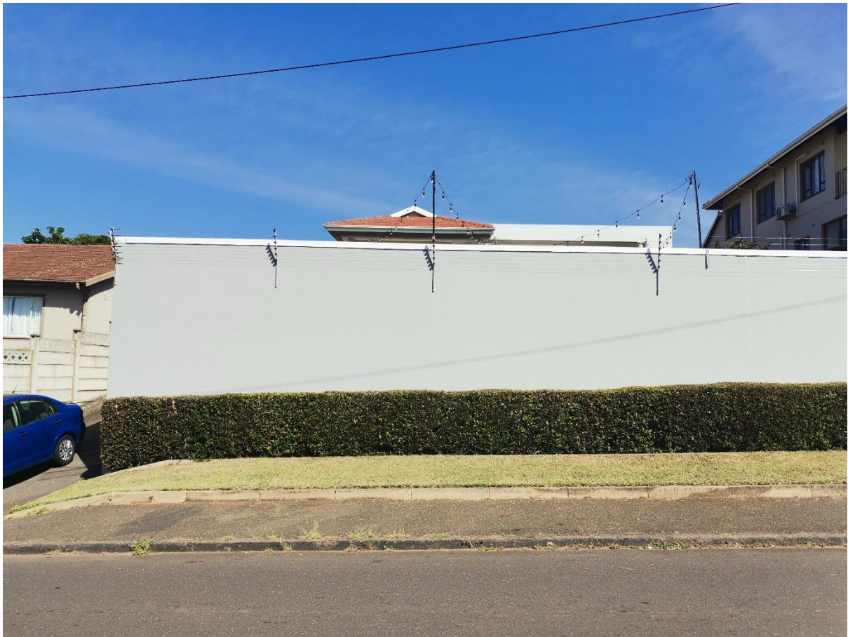
FRONT/EAST ELEVATION FROM ROAD SHOWING EX. BOUNDARY WALL
