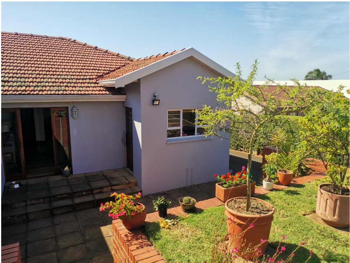
PART WEST ELEVATION/ REAR VIEW OF EX. HOUSE
