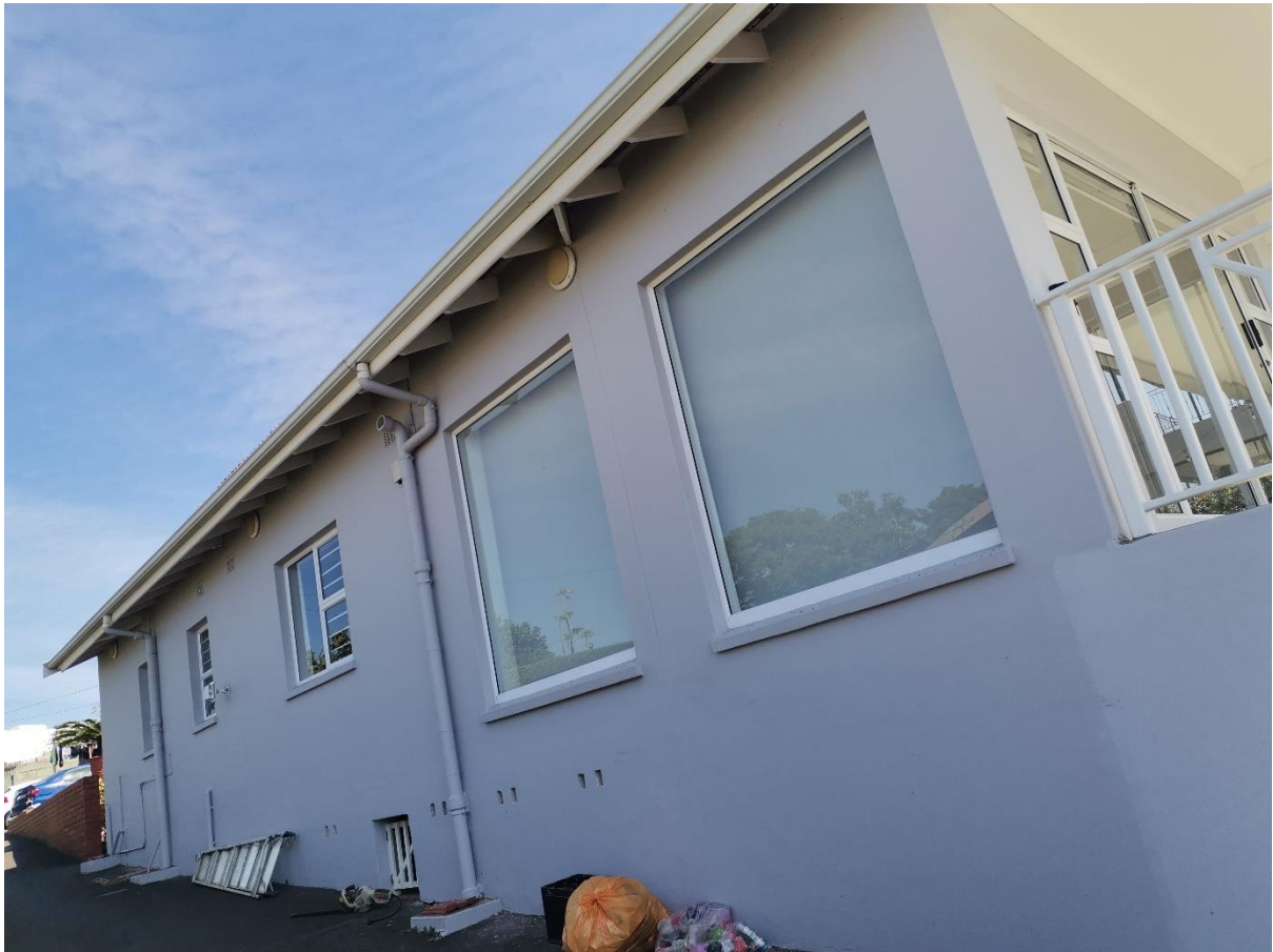
SOUTH ELEVATION LOOKING UP FROM DRIVEWAY
