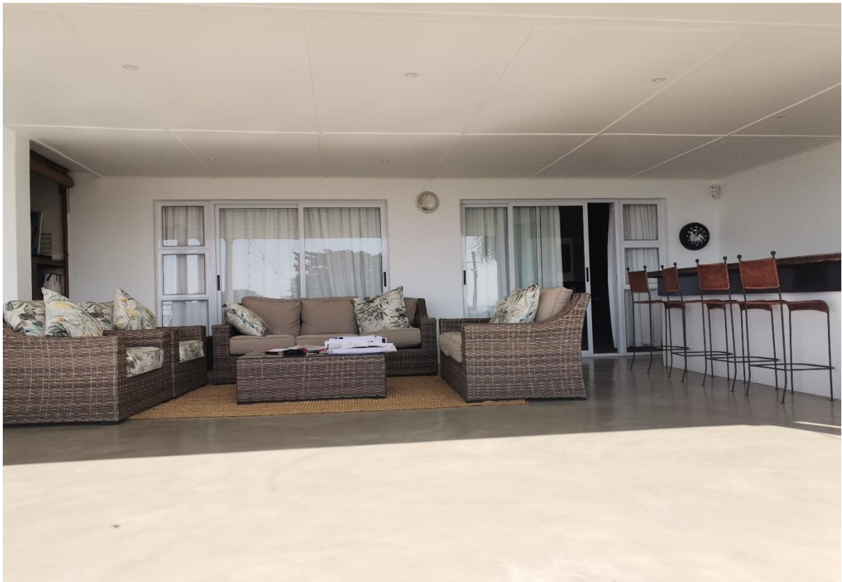
EAST ELEVATION CLOSE UP SHOWING NEW SLIDING DOORS
