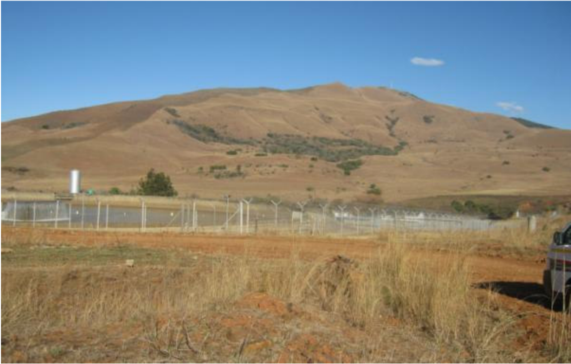
Figure 5 Southerly direction of the Bosloop substation
