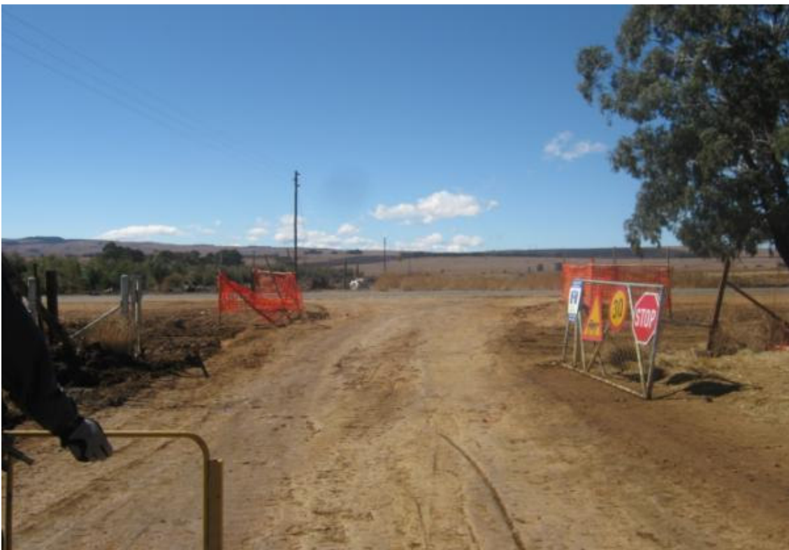
Figure 4 Easterly direction of the Gumeni substation
