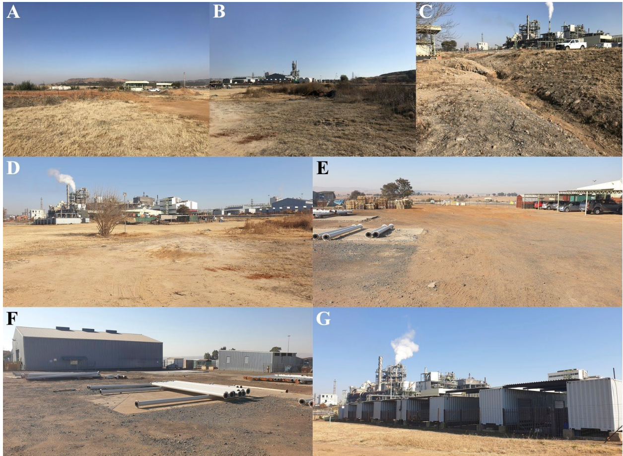
Figure 6: Disturbed nature of the landscape. A: southern part of the property looking south, showing spoil heap stockpiles for backfilling and excavations in the mid-ground; B: southern part of the property looking north, showing extensive on-site facilities in the background and vegetated spoil heaps in the mid-ground; C: southern part of the property with subsurface excavations and no associated archaeological heritage; D: southern part of the property looking west, showing the significantly altered (flattened/terraced) landscape; E: central part of property looking south, showing vehicle and secondary (access) road disturbances to the area; F: central part of the property looking southeast, showing concrete workshop floors and additional on-site buildings; G: central part of the property looking northwest towards the Newcastle Chemical Park, with on-site buildings in the foreground.
