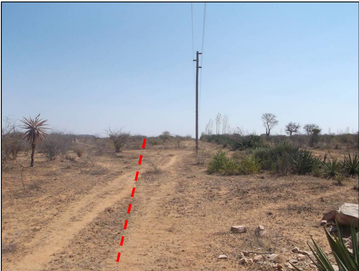
Figure 12: View of pipeline route adjacent to existing Eskom line
