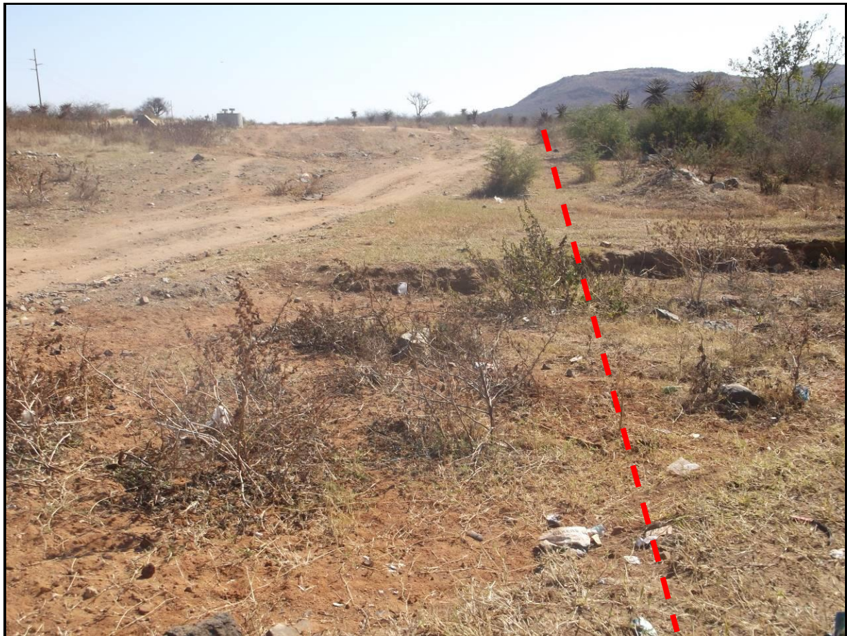
Figure 6: View of pipeline route across the Northern bank of the Rooisloot River.
