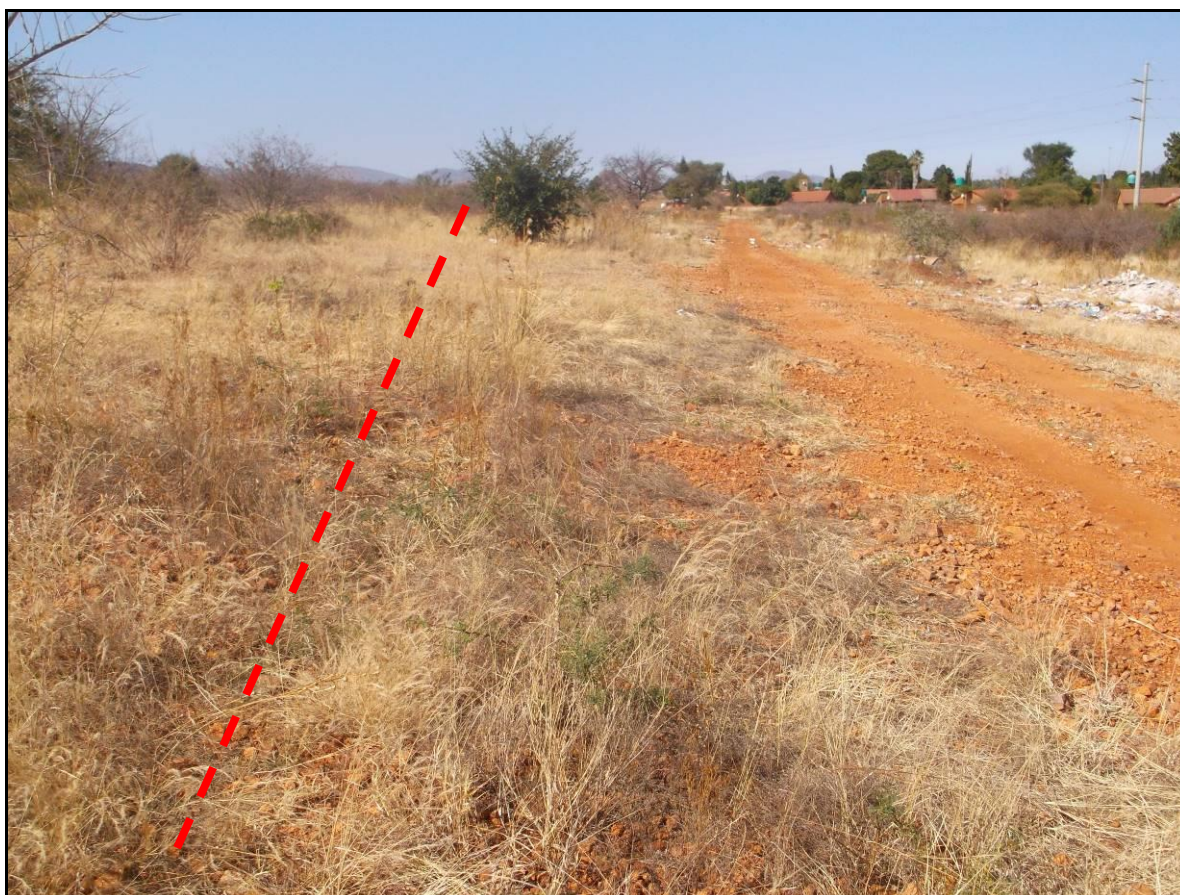
Figure 2: View of proposed pipeline route next to existing pipeline and access road
