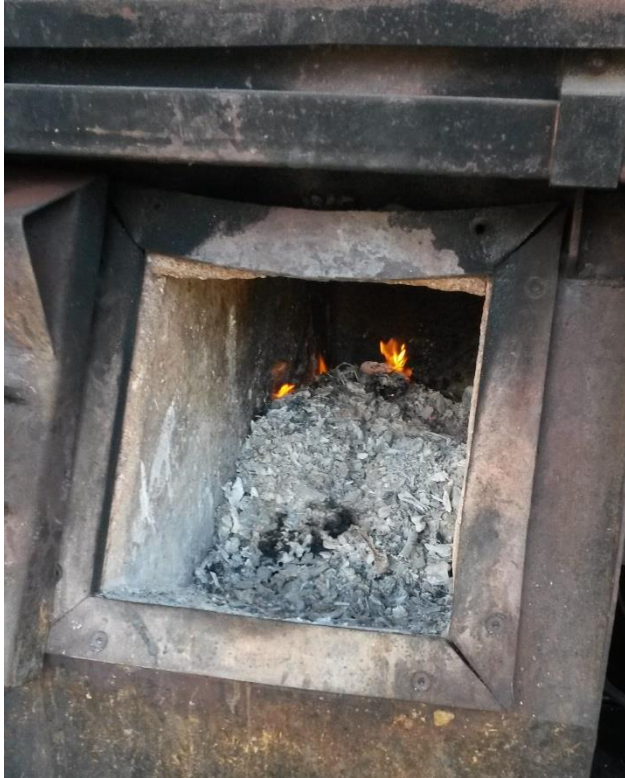
Photo 5: Waste inside the incinerator after incineration
