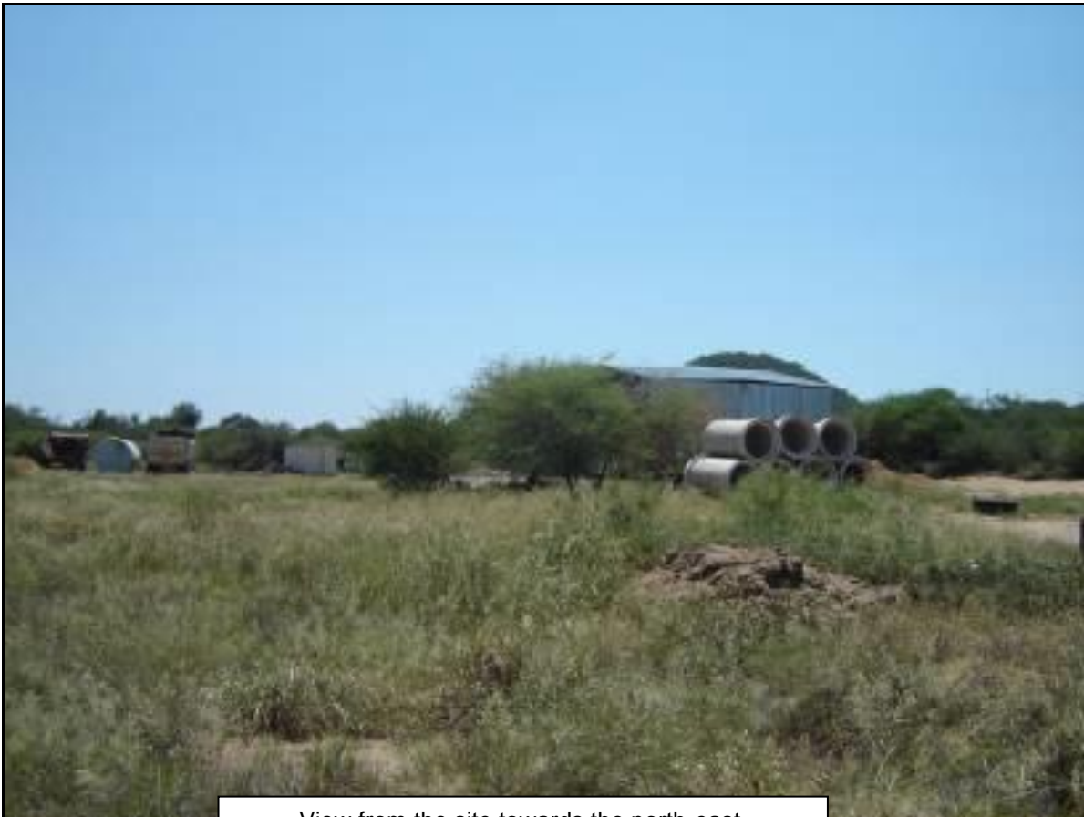
View from the site towards the north-east.
