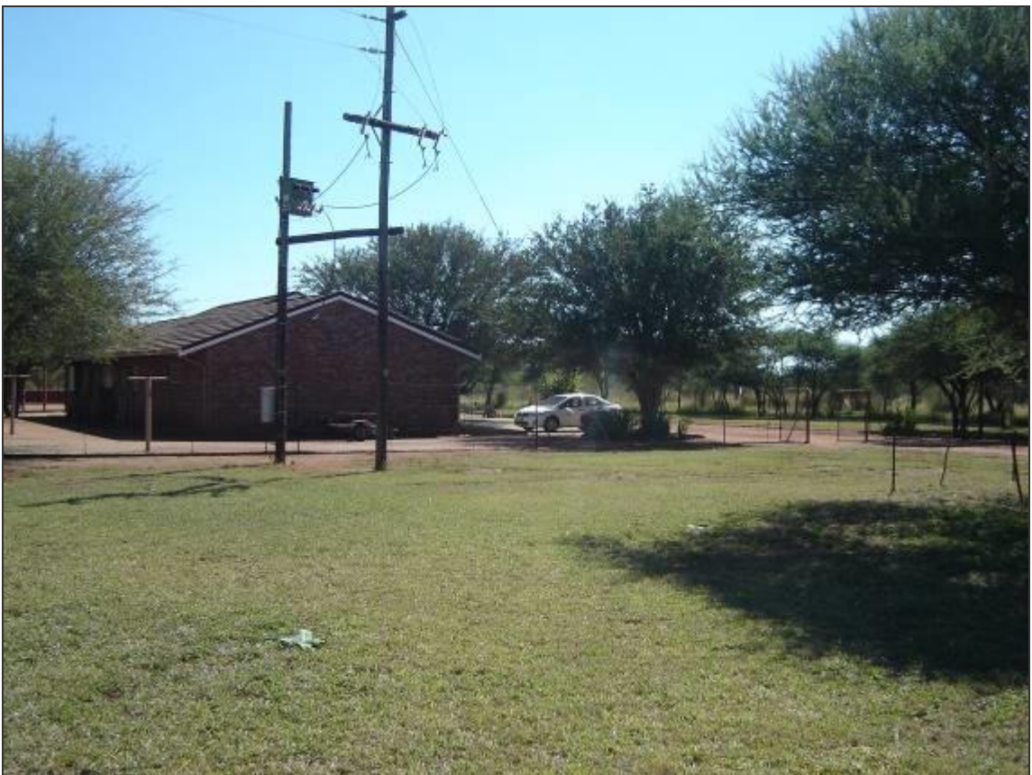
Figure 8: View from the site to the north-west and existing electricity connection point to be used next to the house on the property.
