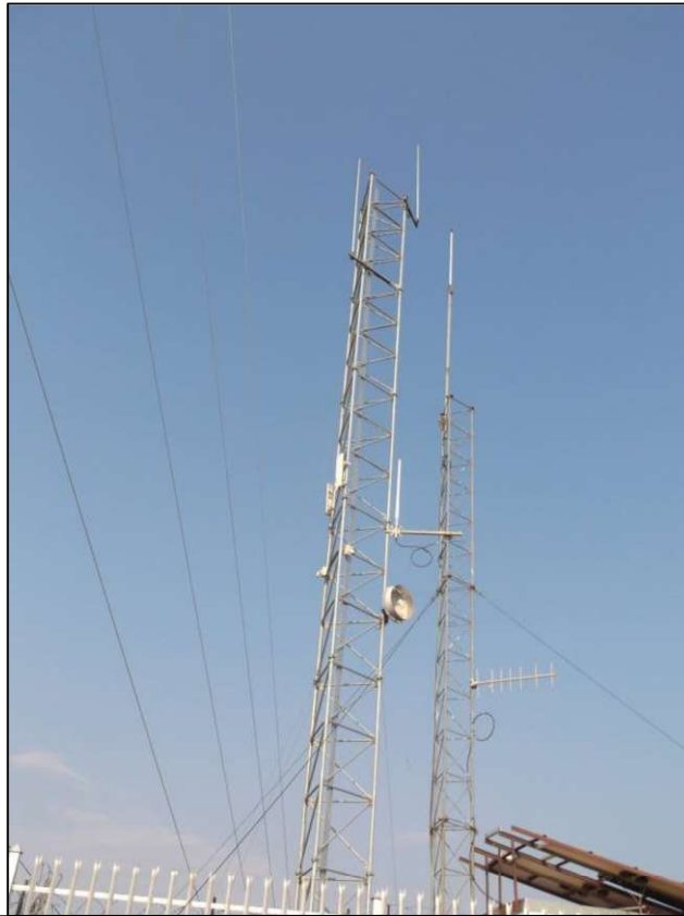
Figure 10: View of existing masts in the vicinity of the site.
