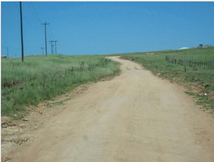
Figure 2-3 Some of the roads in the impoverished areas of the Eastern Cape are in a poor condition and might need upgrading for feedstock transport
