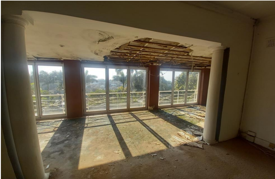
FIG. 7. View from master bedroom to existing balcony
