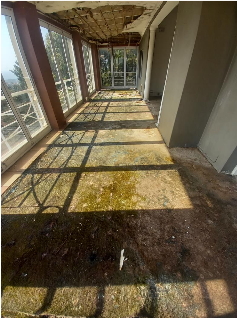
FIG. 8. View of existing balcony
